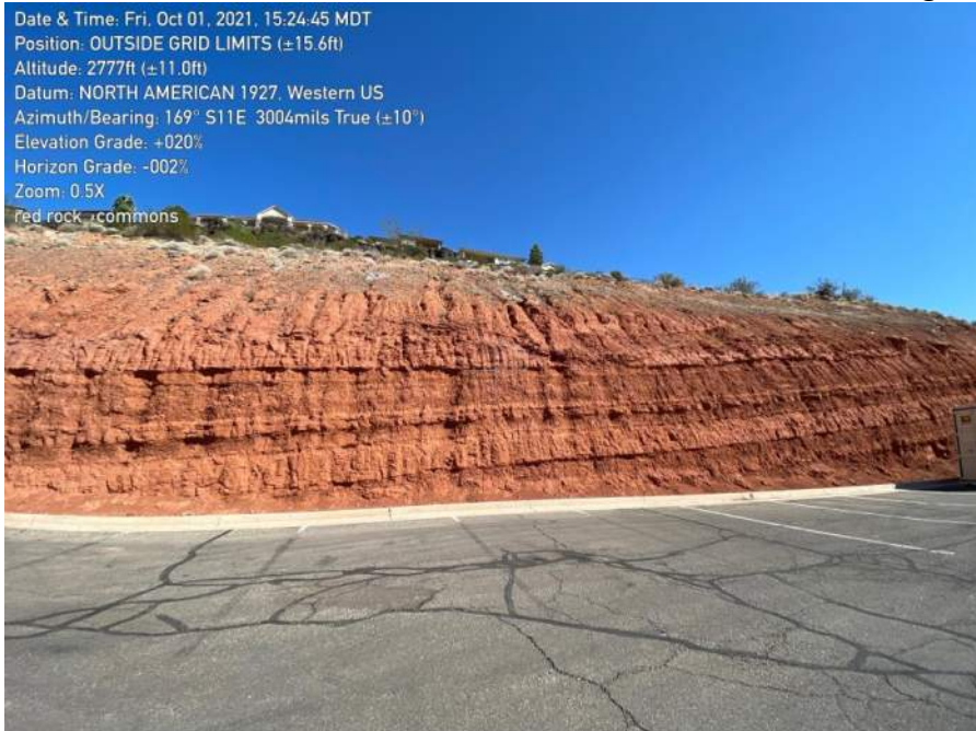
Photo No. 6 – View of cut face in shale bedrock – Red Rock Commons
