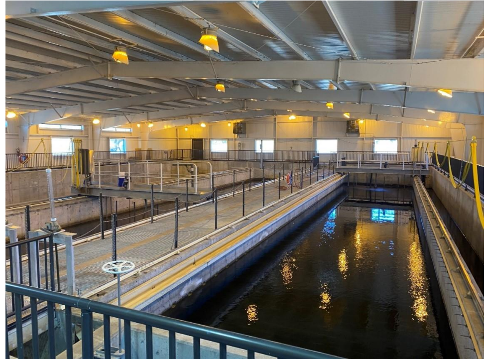
St. George Water Reclamation Facility (WRF)
