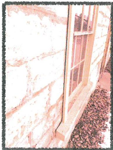
**CAULK EXISTING WINDOWS AND DOORS AS REQUIRED.** For long-term protection, caulking of these surfaces would be an excellent idea at this point. Backer rod should be used so the thickness of caulking is limited to  $1/4$ " to  $1/2$ " and a quality sealant such as Sika Sikaflex 15LM should be used. (Free shipping on order over \$100)
