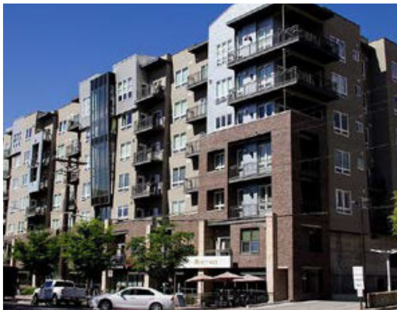
Figure 6.7 (1). Example of Livable Balconies.
