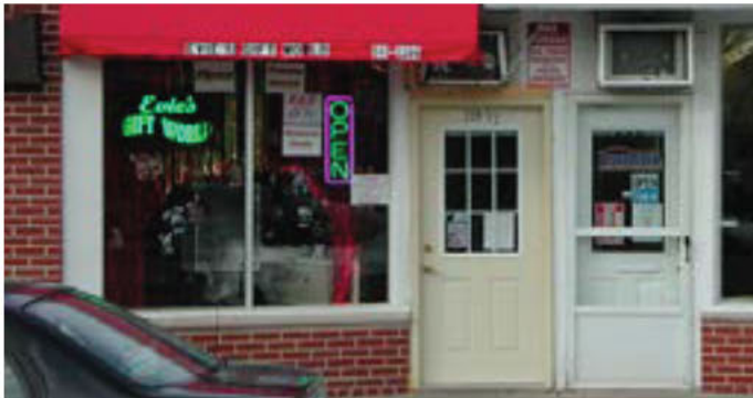
Prohibited: Residential Grade Doors on Commercial Buildings.
