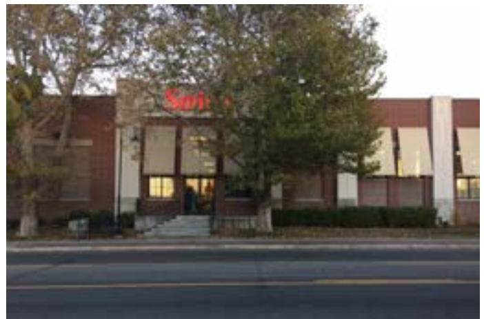
Figure 7.6 (1). Screening of Buildings.
