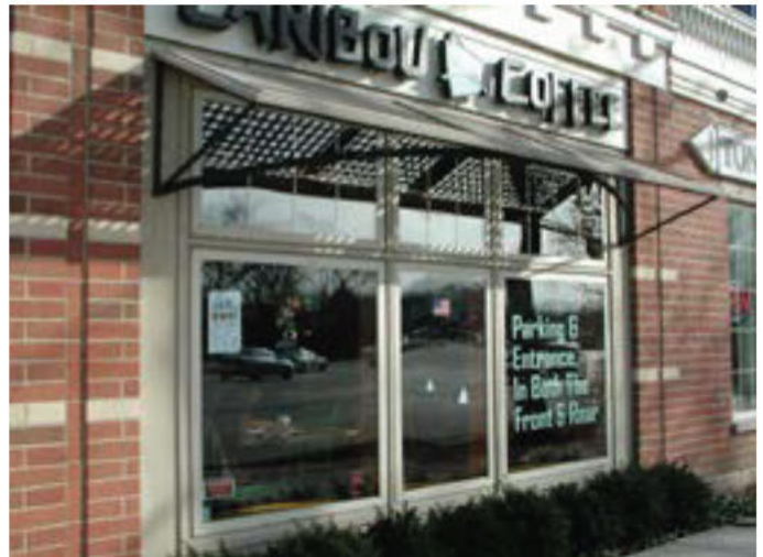
Permitted Awnings: Metal
