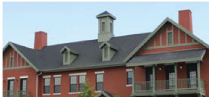
Roof Materials: Asphalt Composite Shingles
