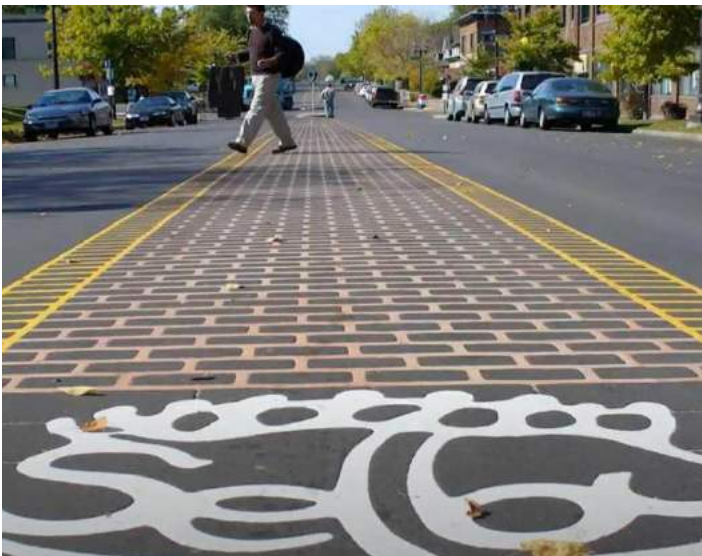
Example of thermoplastic high-visibility crosswalk (Source: Ennis Flint)
