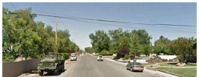
100 N between 100 E and Main Street where there's curb and parallel parking
