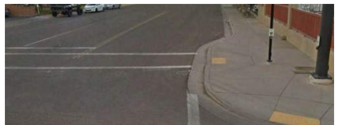
Existing curb bulb-out on 300 W and State Street, Hurricane, UT (Source: Google Street View)
