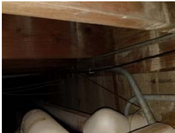
Photograph 16 – 2x4 ledger supporting floor joists.
