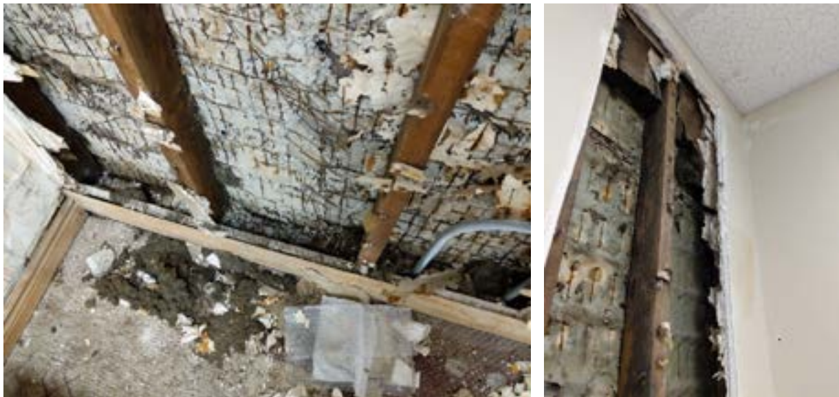
Photograph 10 – Perimeter wood stud walls exposed on the North (left) and South (right) perimeter walls were excessive water damaged was observed.
