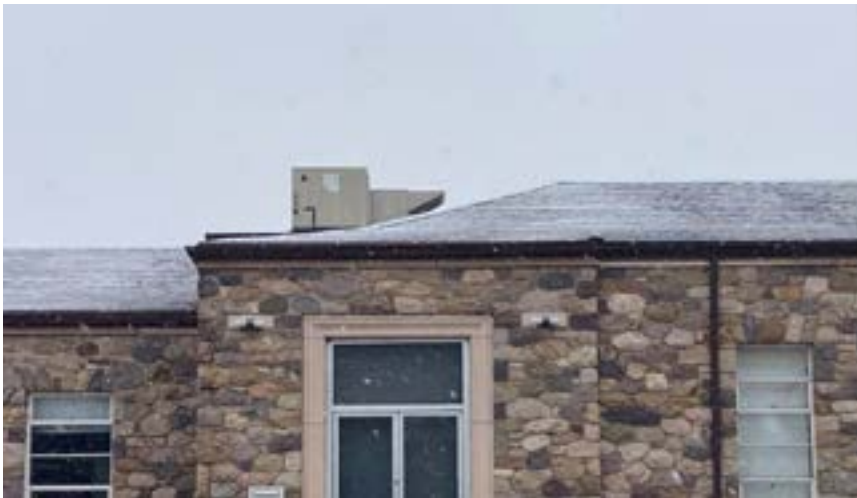
Overbuilt roof showing flare to front of cast concrete coping.
