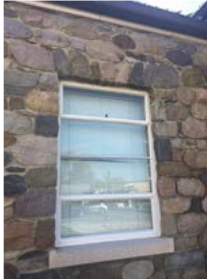
Original steel window and cast concrete sill.
