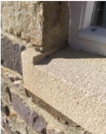
Original steel window and cast concrete sill.
