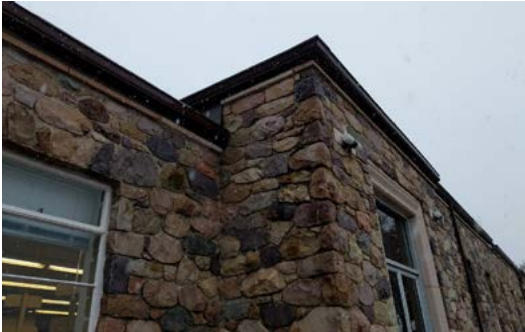
Photograph 4 – Reentrant Corner on North-West side (South-West side similar)
