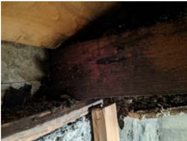
Photograph 7 – Roof truss bearing on sill plate at top of stone wall in mech room (special case) More commonly bearing on interior stud wall. Left: Observed in coal storage room with precase cap beyond, Right: Observed east of attic access
