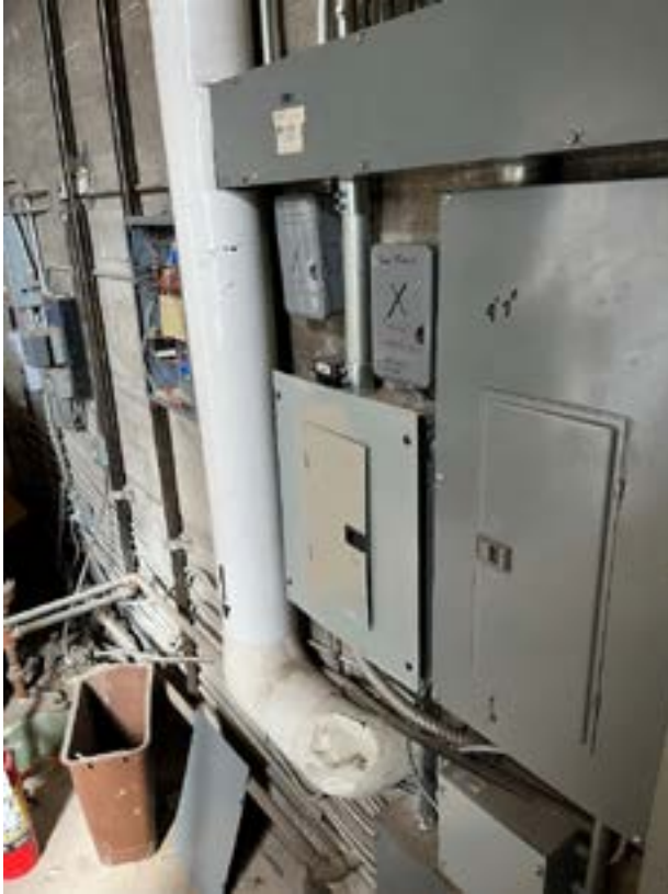
Panel with plumbing piping running underneath.
