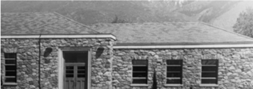
Early image depicting west elevation cast stone coping.
