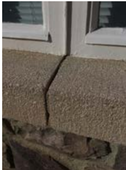
Original steel window and cast concrete sill.
