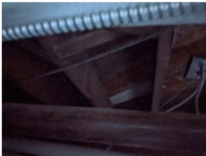
Photograph 17 – Diagonal 1x floor sheathing
