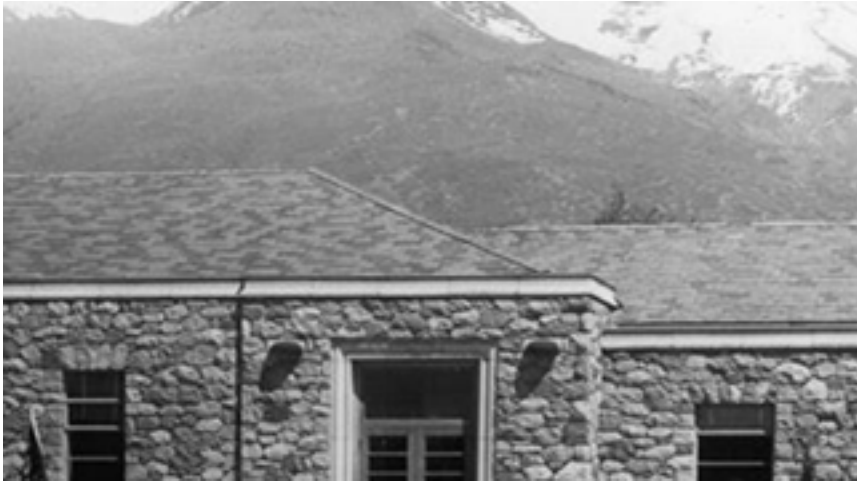
Original roof shown framed behind cast concrete coping.
