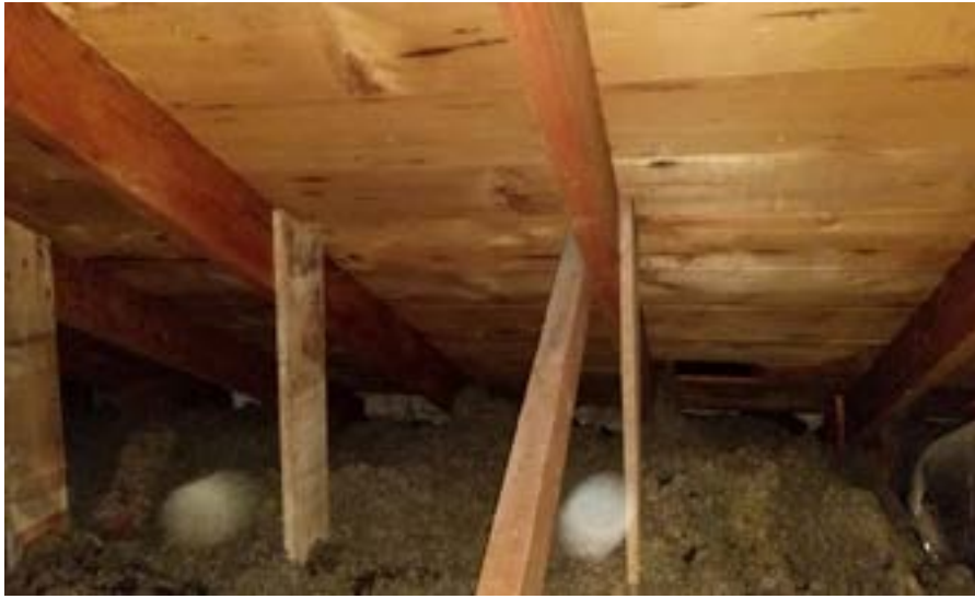
Photograph 6 – Straight 1x Roof Sheathing
