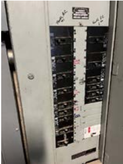
Existing 3 phase, 120/240V high leg panel
