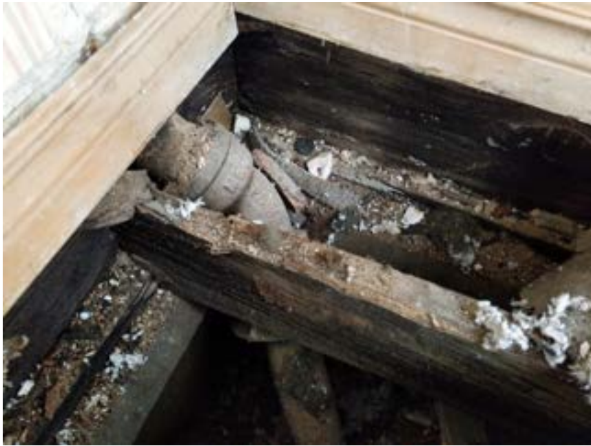
Photograph 17 – Main floor joist bearing condition at corner
