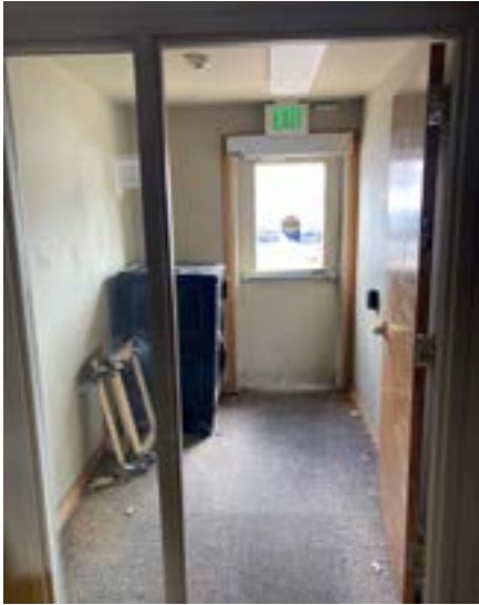
East entry door. Note lack of clearances on the strike side of the door.
