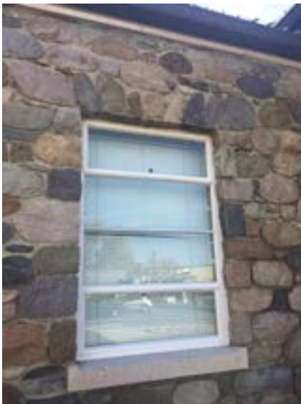
Keystone lintel on west elevation.
