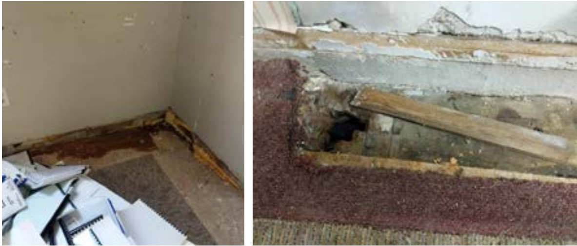
Photograph 11 – Damage to main floor system observed in North-East corner (left), North region (right) and other locations throughout building where water intrusion has occurred.
