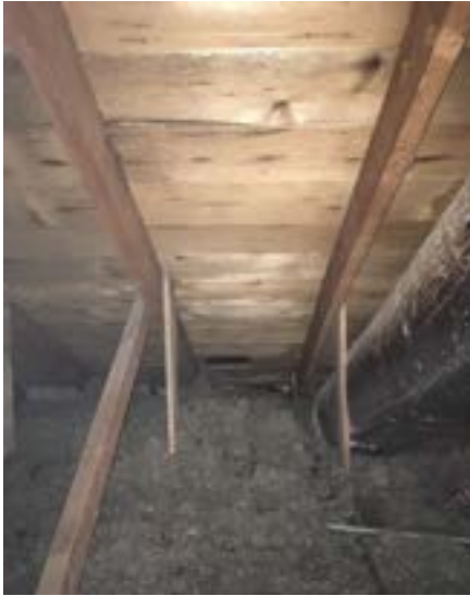
Existing trusses in attic.
