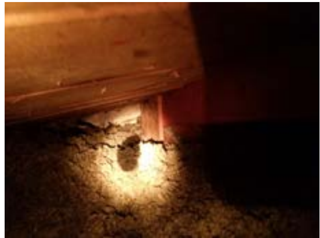
Photograph 7 – Roof truss bearing on sill plate at top of stone wall in mech room (special case) More commonly bearing on interior stud wall. Left: Observed in coal storage room with precase cap beyond, Right: Observed east of attic access
