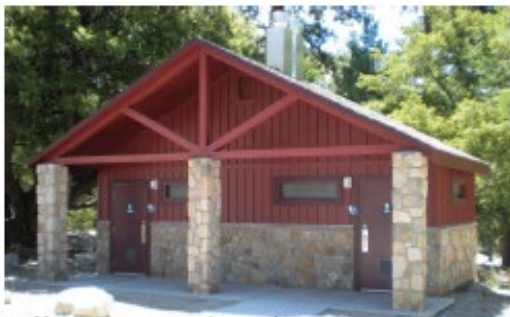
Prefab restroom structure (Or match Legacy)
