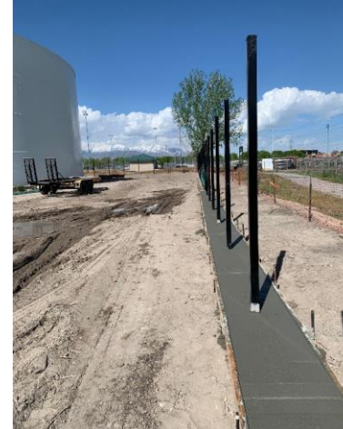
Installation of powder coated fencing along west side of property
