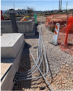
Electrical conduits from pig launch vault to electrical building
