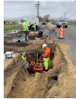
12-inch gate valve installations
