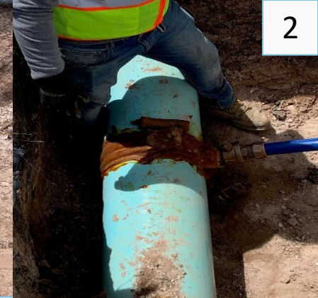
Applying wax tape and poly-ply wrap to 12"x2" brass saddle
