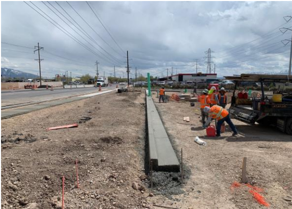
Sidewalk and curb and gutter installation
