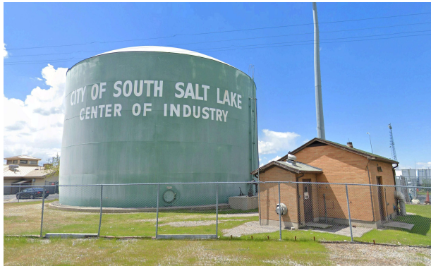
Main Lift Station 2250 South 600 West
