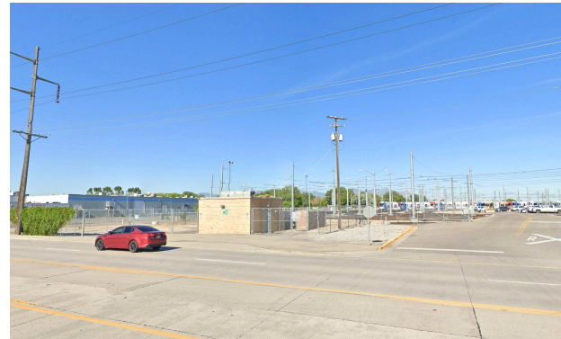
Pump House Lift Station 2280 South 900 West
