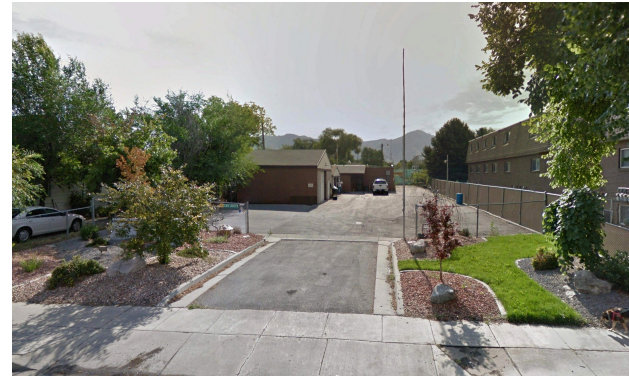
Well Complex 2501 South 300 East
