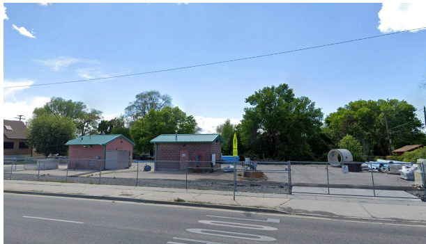
Well Complex 3190 South 700 East
