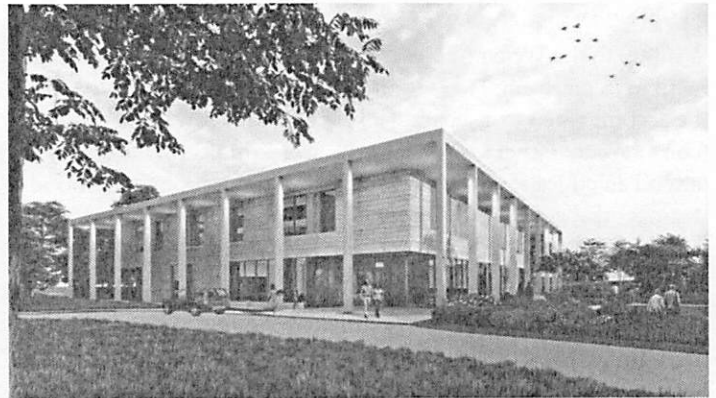
Above: The new Lakewood Welcome Center Building
