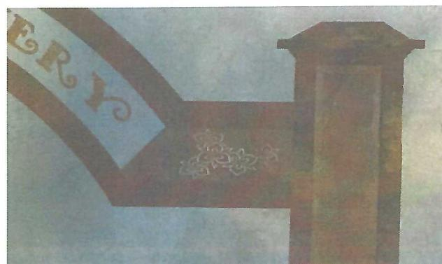
The design is intended to oxidize and patina. The rusting coloration is made uniform by sand blasting the surfaces and letting the oxidation progress at the same rate. Its stout construction and designed weeping holes allow water to shed and not collect and freeze, thus reducing the risk of freeze bursting with cold weather.
