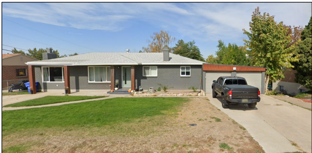
Street View, Looking North
