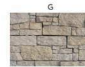
G RUBBLE LIMESTONE WALL DRY-STACKED
