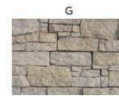
G RUBBLE LIMESTONE WALL DRY-STACKED
