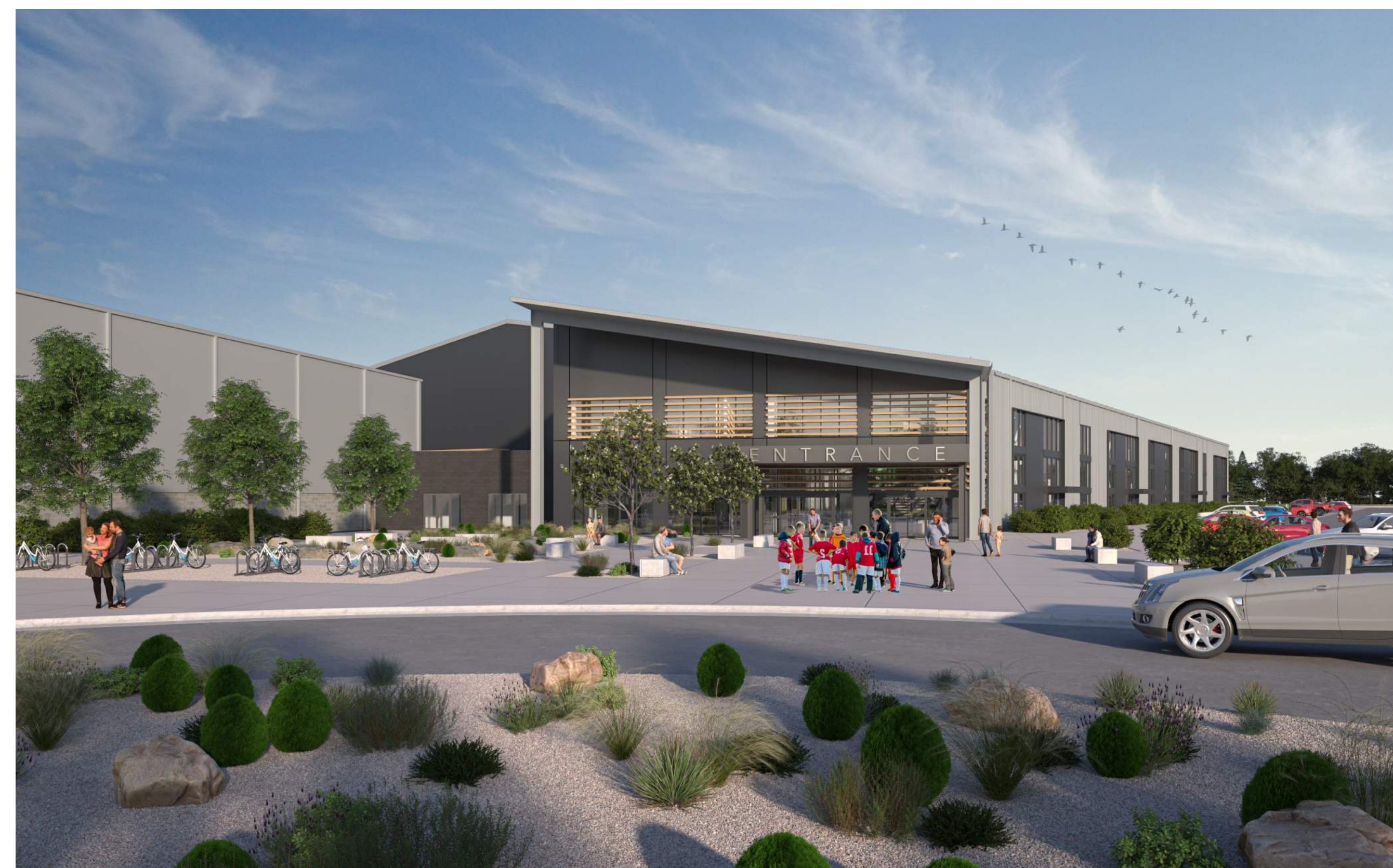
VIEW OF MAIN ENTRY FROM CIRCULAR DROPOFF ZONE
