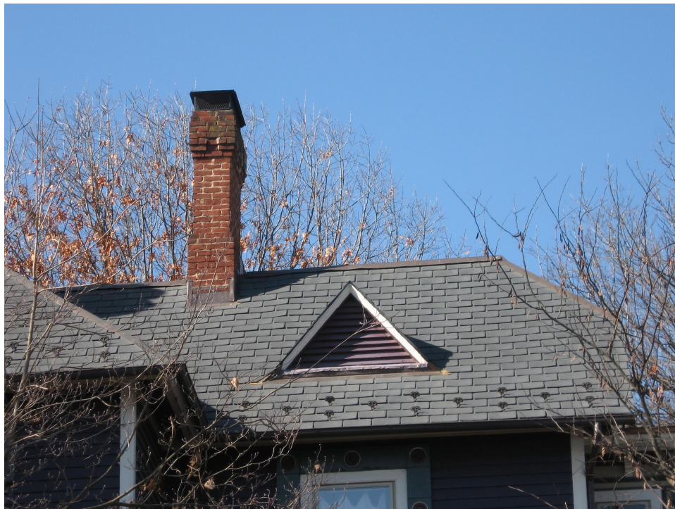
Example of a synthetic slate roof in a Roanoke, Virginia historic district.
