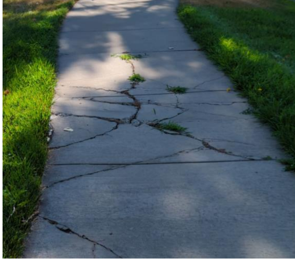
MULTIPLE CRACKS
