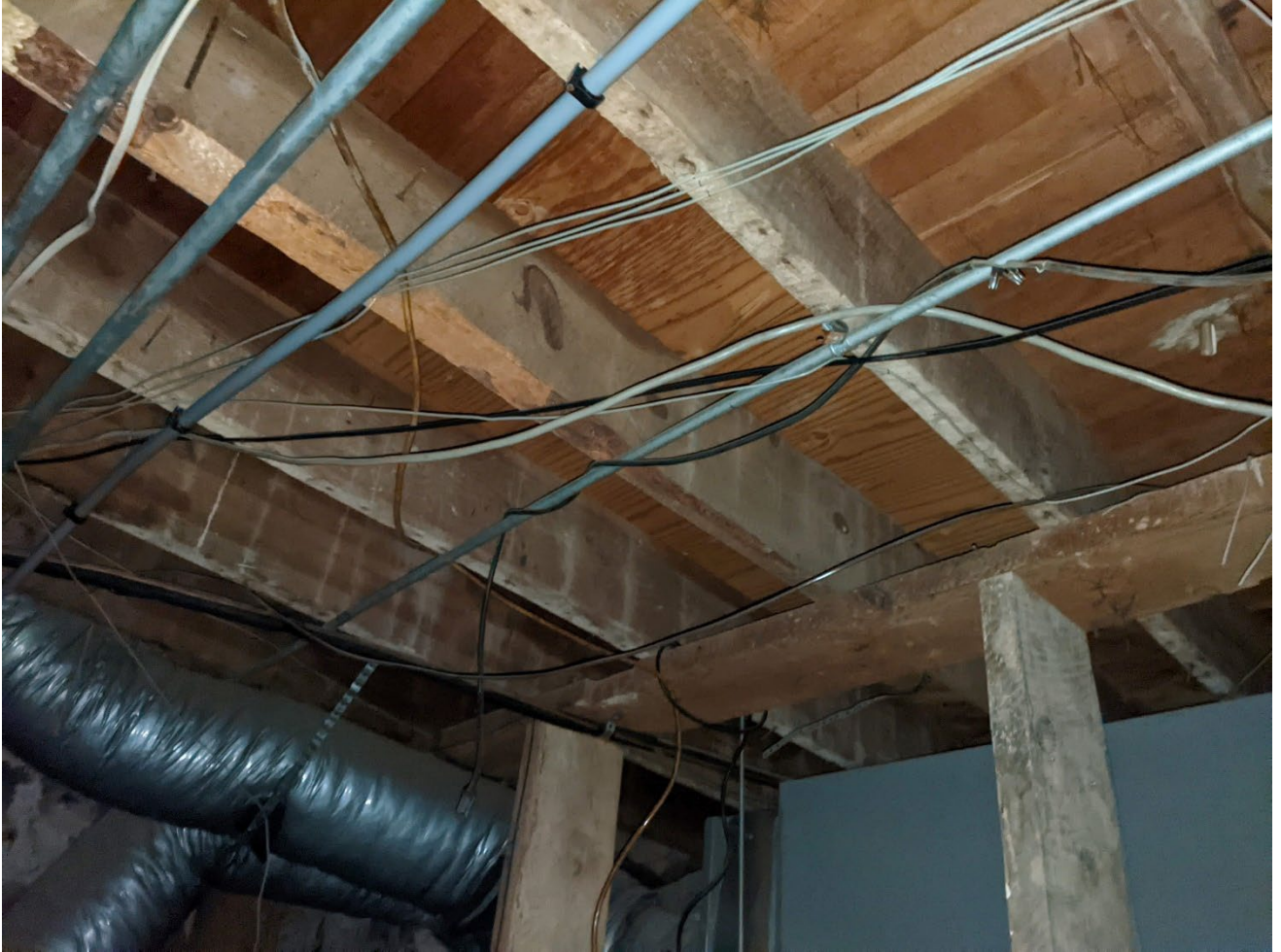
Existing floor joists with subfloor above
