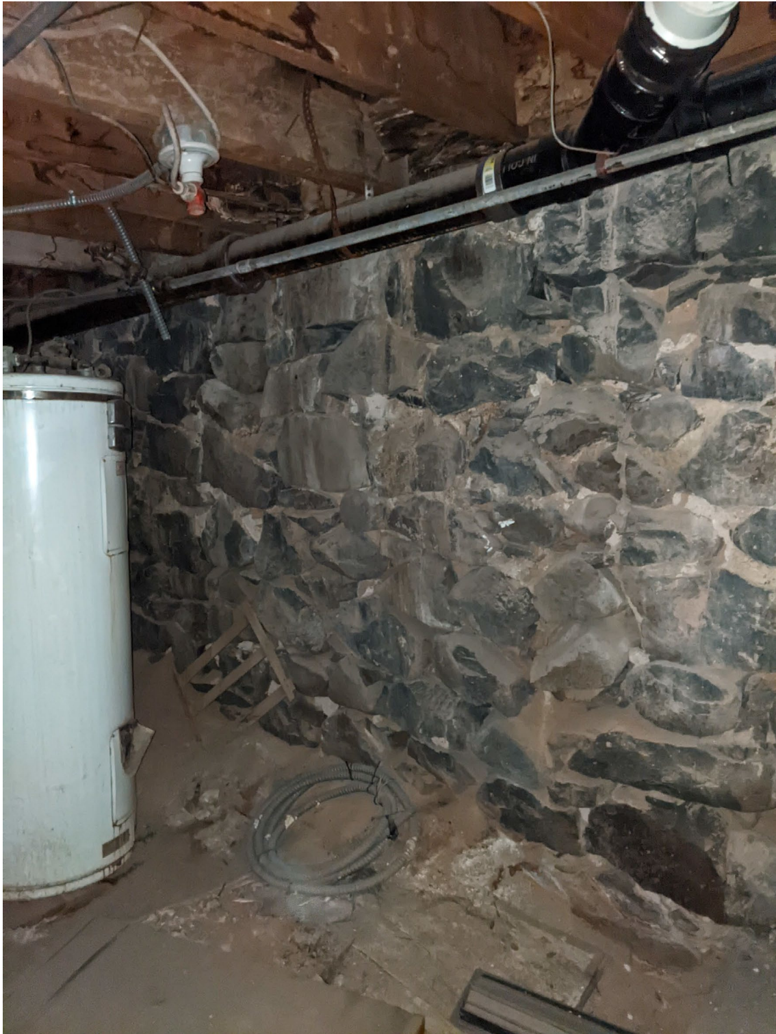
Stacked stone foundation wall
