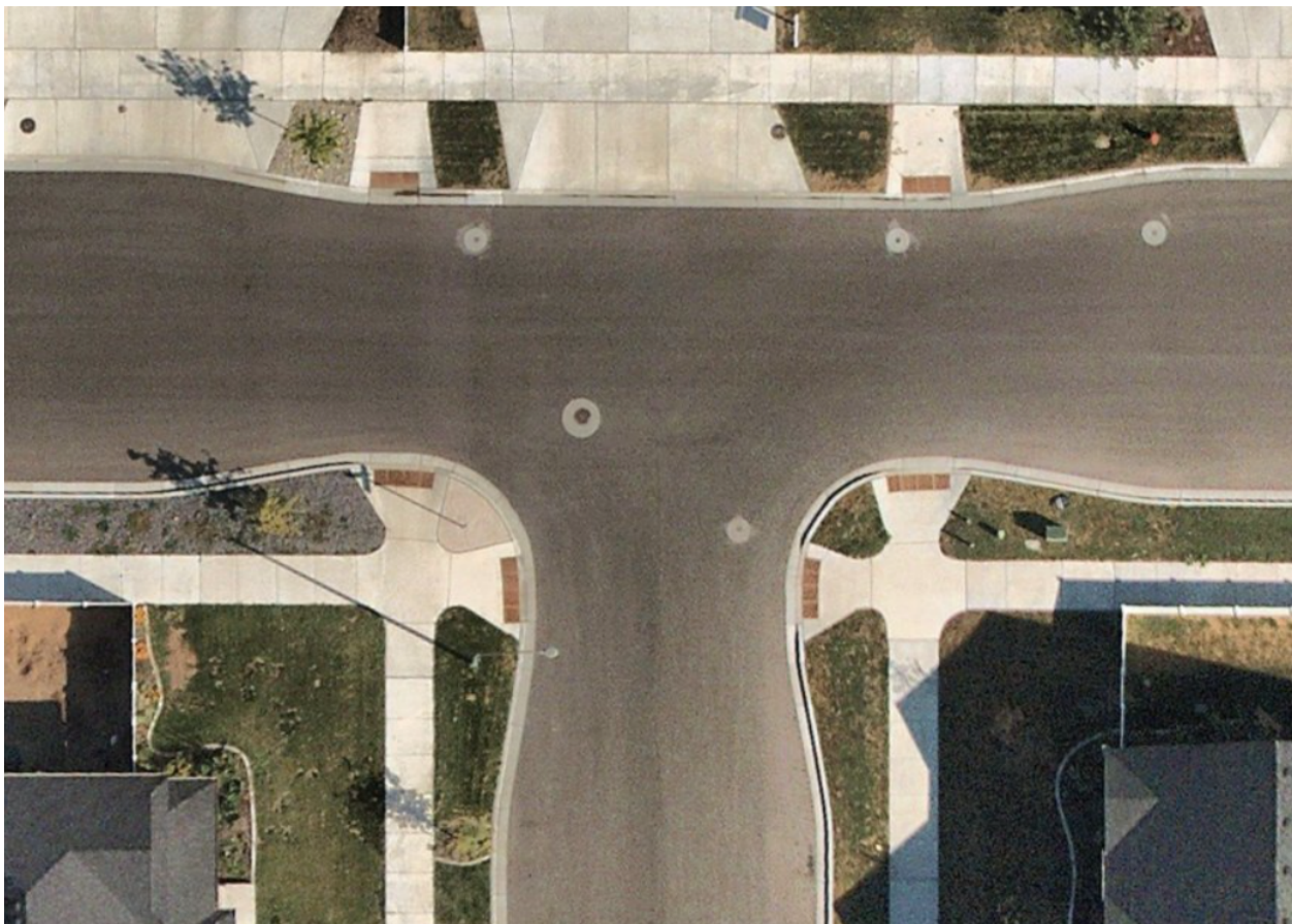
Figure 6: Bulbouts at a local street T-intersection in Provo
