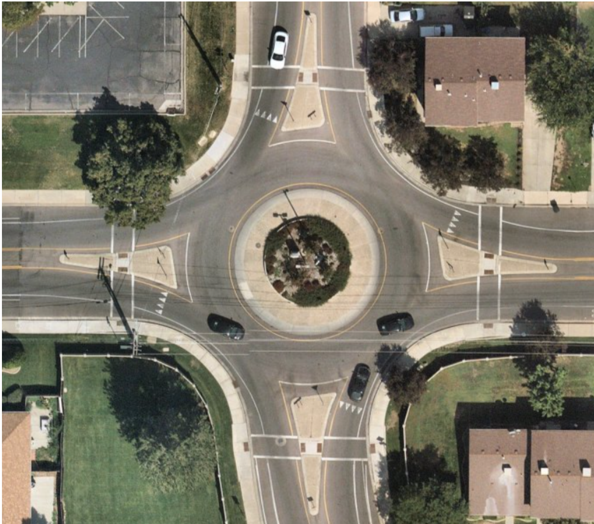
Figure 4: Roundabout at the intersection of two collector roads in Provo
