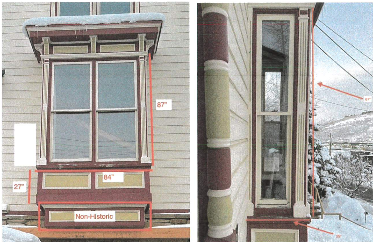
Figure 3: Measurements of Bay Window from the front and side.
