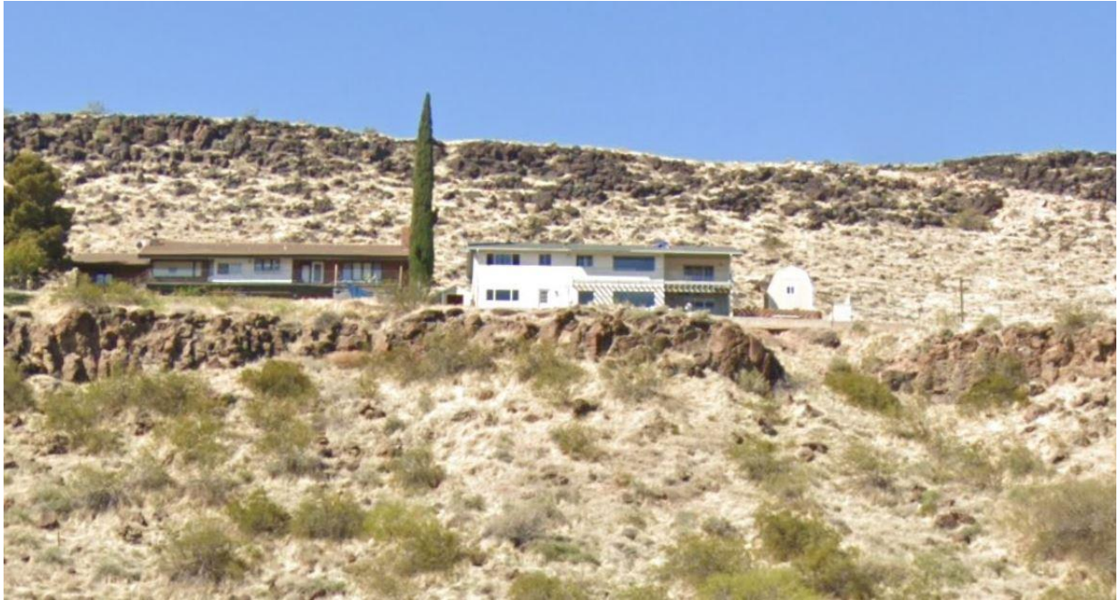
Rear of House – Before
