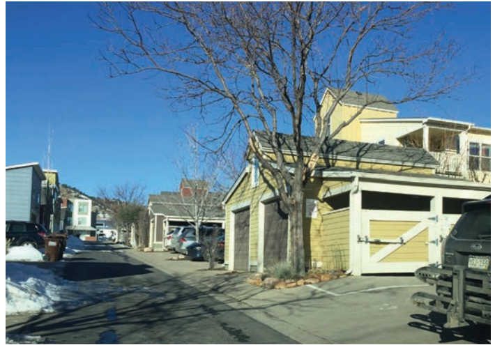
An alley with flat concrete edge with concrete head-in parking spaces that employs several landscape islands.
