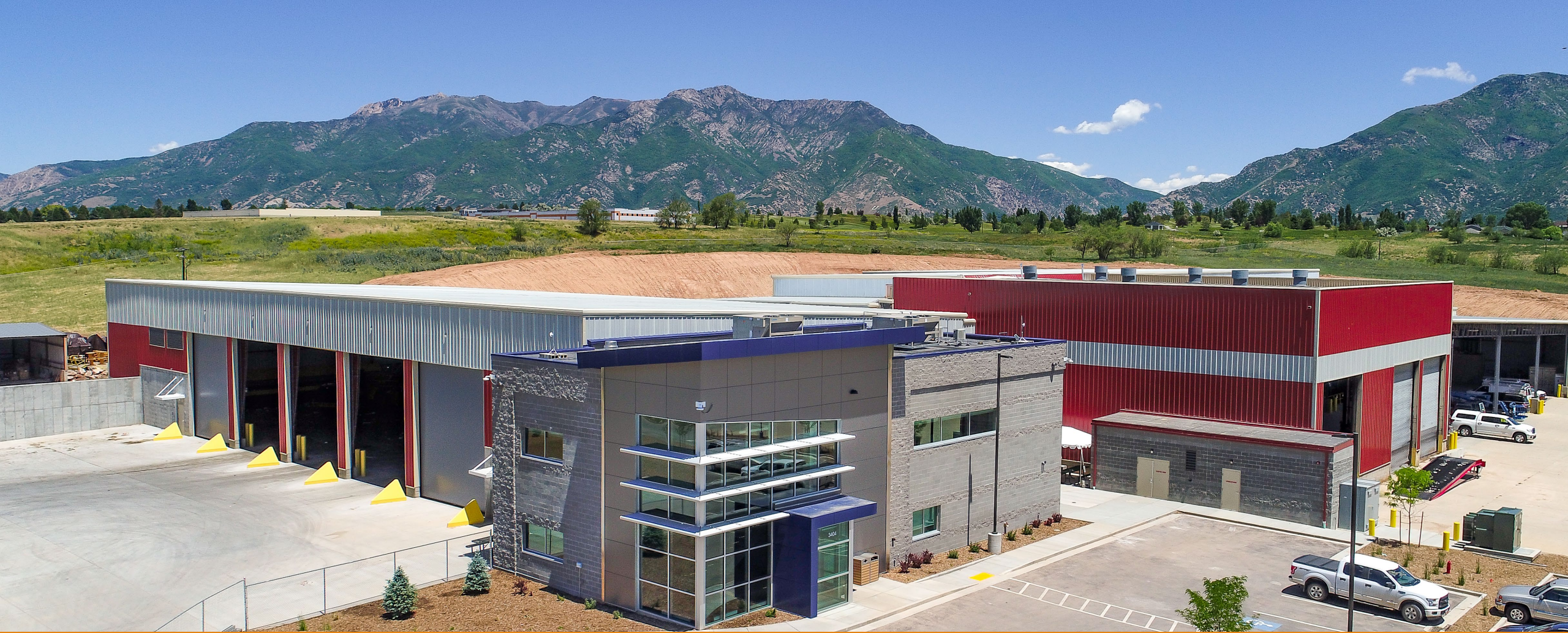
Davis Material Recovery and Transfer Facility
