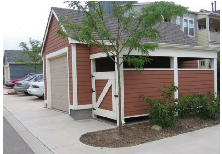
Flat concrete edge allows employment of landscape islands easily. The small ornamental trees that can grow in these islands reduces the formation of heat islands significantly.
