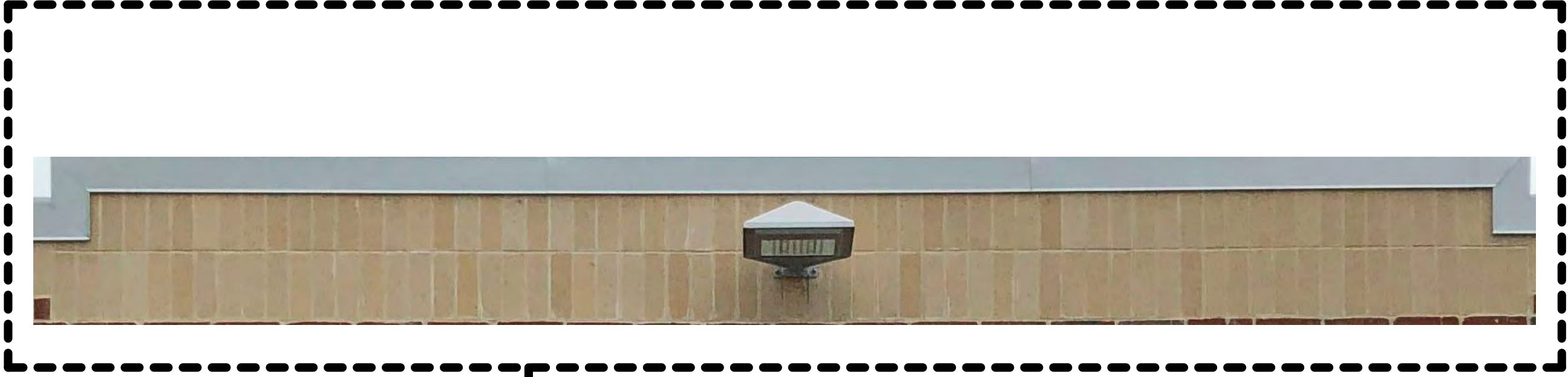
RAISED PARAPET AT ENTRY (BRICK COLOR #2 ACCENT)
