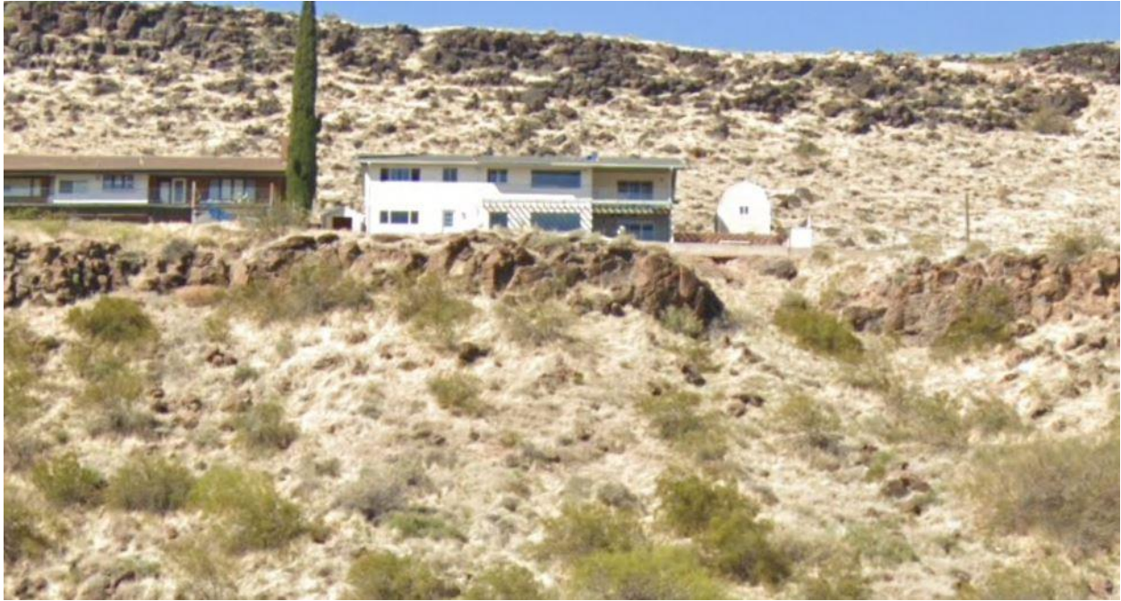
Rear of House – Before
