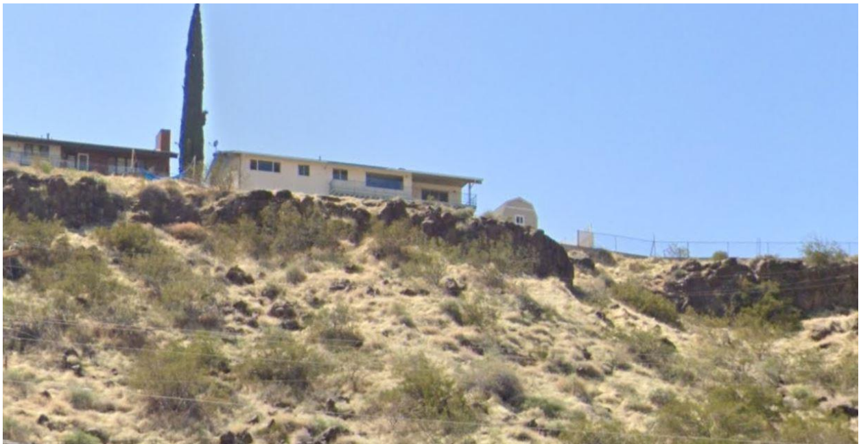
Rear of House - Before
