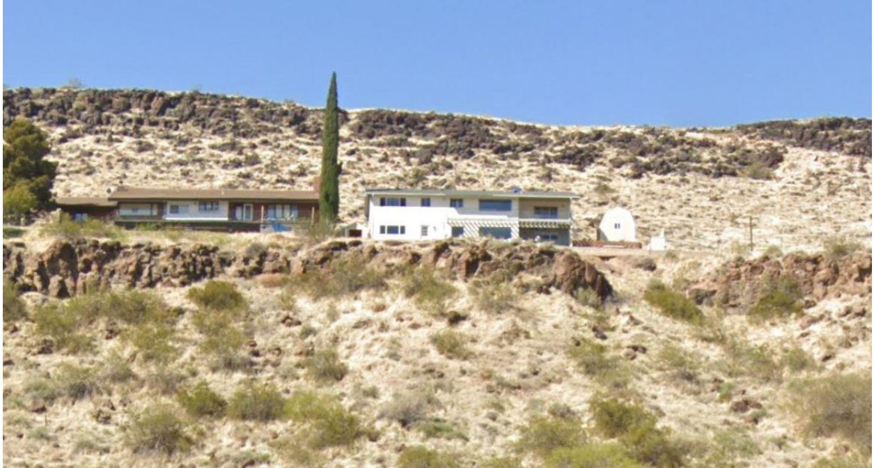
Rear of House – Before
