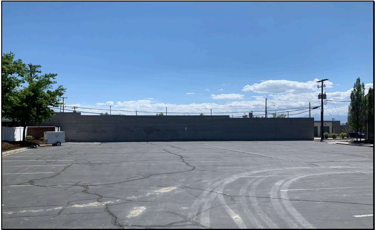
Southerly View of East End
