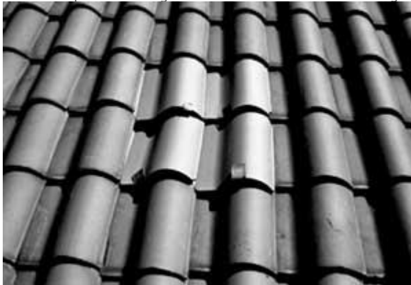
Repairs on this pantile roof were made with new tiles held in place with metal hangers. Photo: NPS files.
