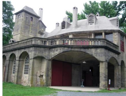
[9] Distinctively-shaped roofs are important in defining the historic character of these early 20 th -century structures: (a) an asphalt shingle roof on a house; (b) and a concrete roof on Forthill, Doylestown, PA (1908-1912), designed and built by Henry Chapman Mercer.
