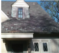
[8] Regular maintenance includes removing leaves that can clog gutters and cause water damage to the exterior and interior walls of a house.
