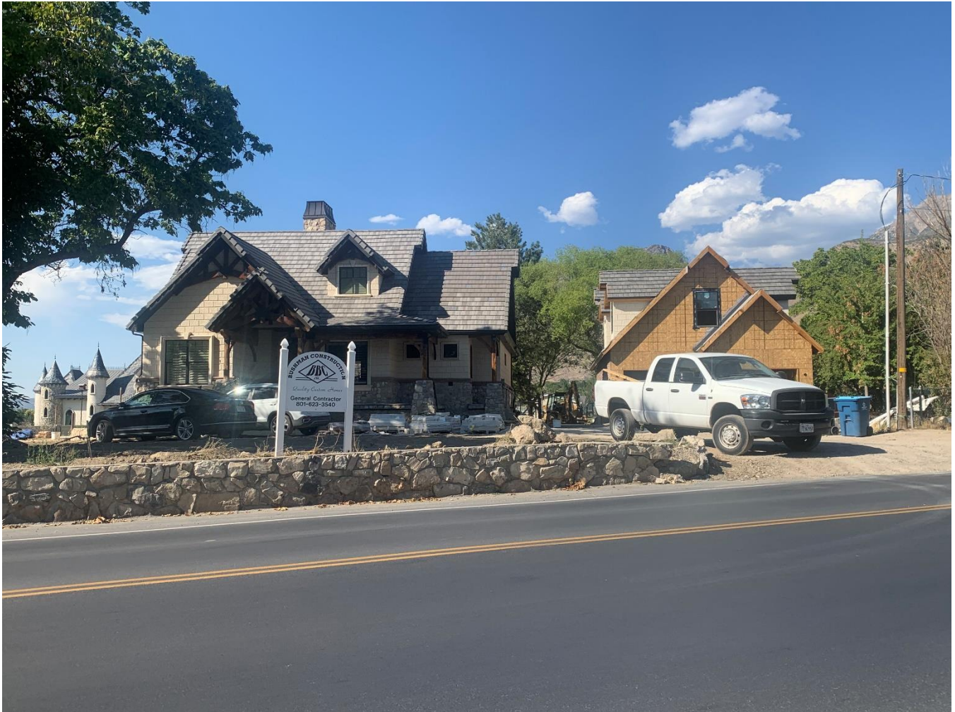
Exhibit 3: New Residential Home Under Construction
