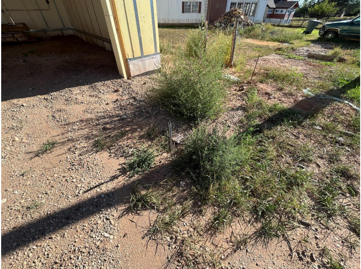
Utilities on East side
