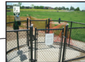
Double gate entry systems (4 Entries)
