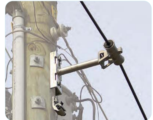
Standoff Bracket with AFL ATGN Single Trunnion
