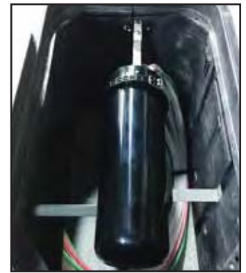
90° Splice closure mounting
