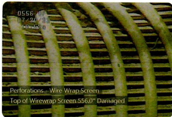
Perforations - Wire Wrap Screen | Top of Wirewrap Screen 556.0" Damaged
