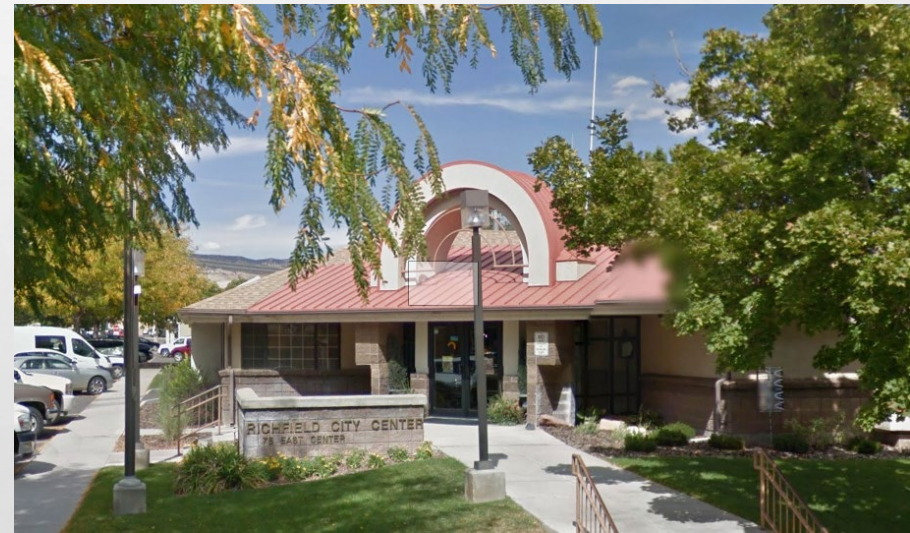
RICHFIELD CITY COUNCIL
