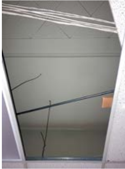
Original ceiling condition.
