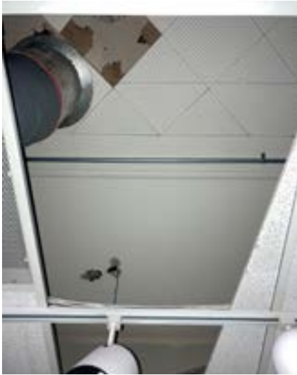
Original ceiling condition.
