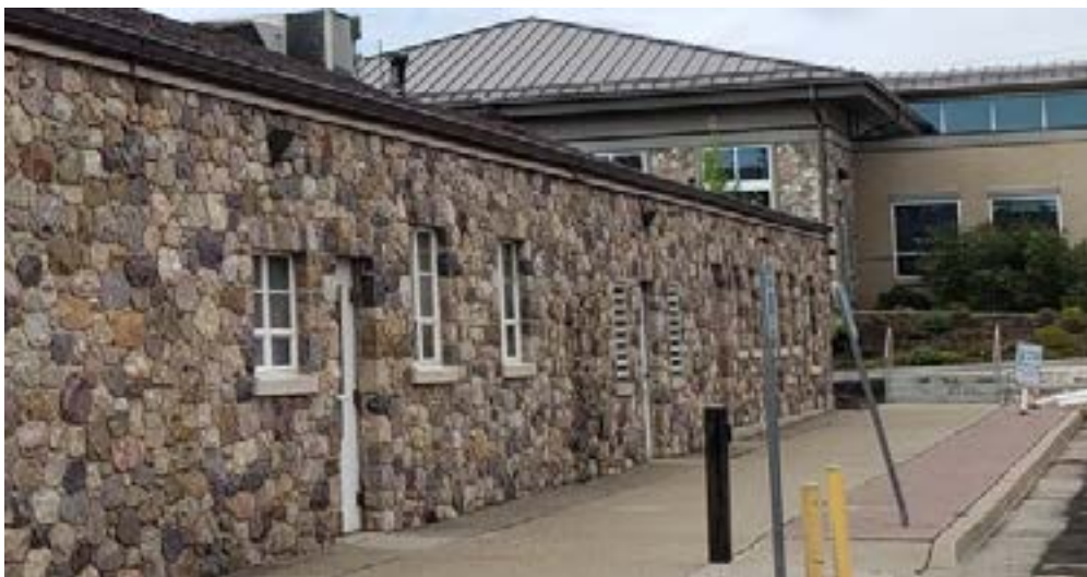
Photograph 3 –East Exterior of Building
