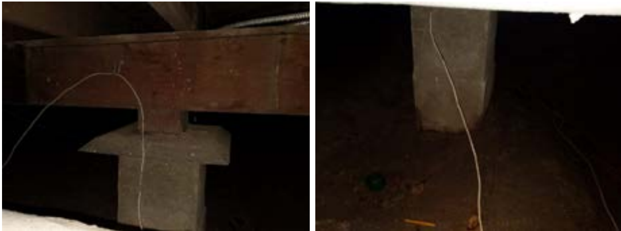
Photograph 15 – Multi-ply 2x support beam in crawl space supporting joist and supported by post. Left: top of post, Right: shovel formed concrete footing
