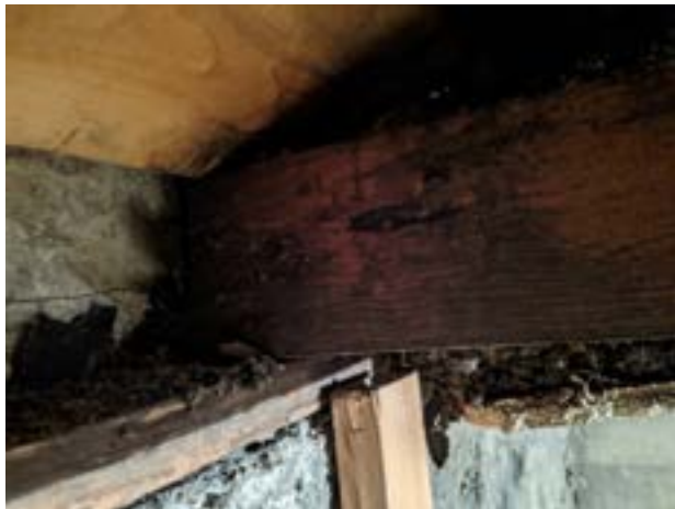
Photograph 7 – Roof truss bearing on sill plate at top of stone wall in mech room (special case) More commonly bearing on interior stud wall. Left: Observed in coal storage room with precast cap beyond, Right: Observed east of attic access
