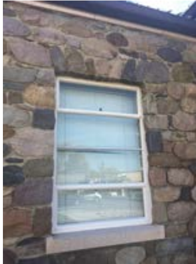
Original steel window and cast concrete sill.
