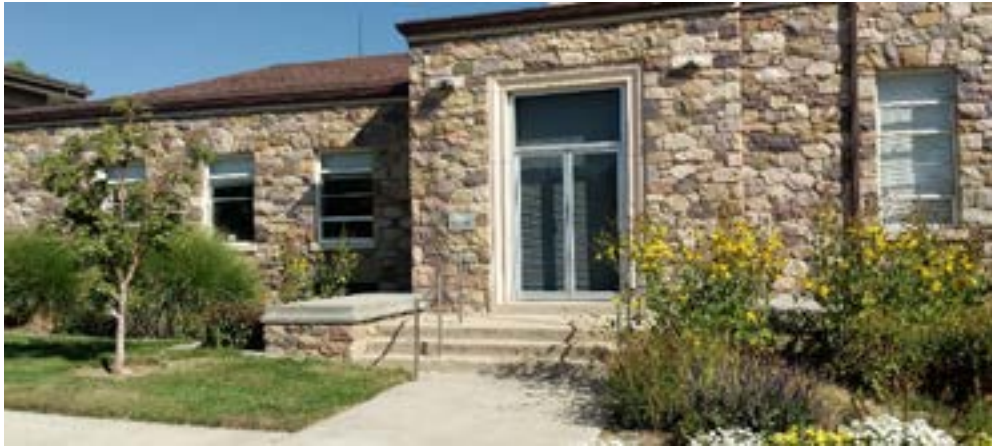
Photograph 1 – North-West Exterior of Building
