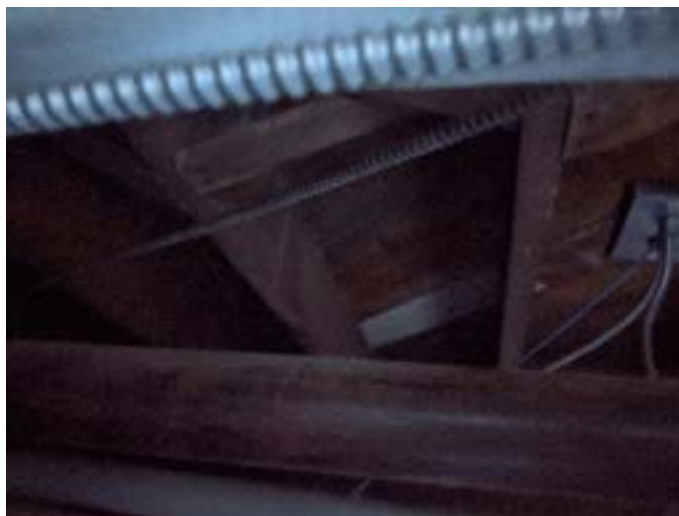
Photograph 17 – Diagonal 1x floor sheathing
