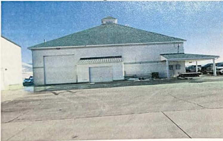
Main Building - Easterly view
