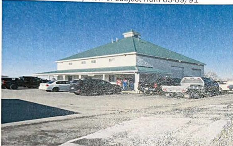
Main Building - Northwest view
