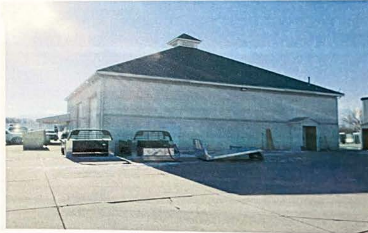
Main Building - Southerly view
