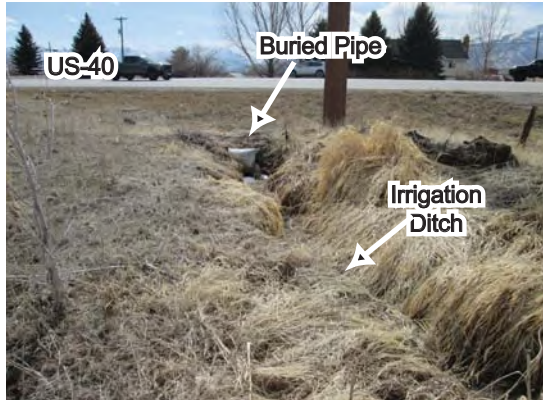
Photo 17. Southwest view at southwestern boundary of Project Area showing irrigation ditch draining into a buried pipe. No water was in the ditch at the time of the March 10, 2021 site inspection.
