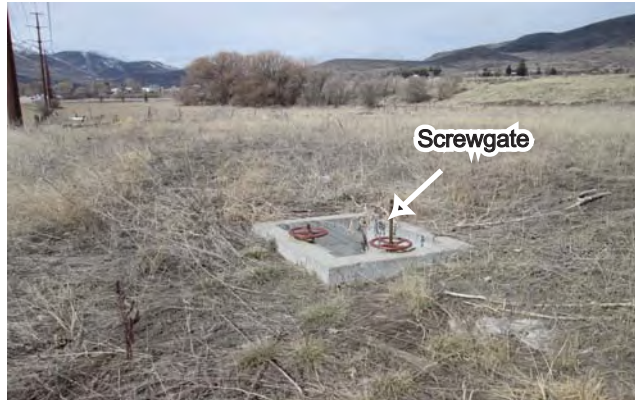
Photo 19. North view of irrigation screw gate observed in uplands located in the southwest corner of Project Area. The man-made irrigation ditch has been placed in a buried pipe to this control box location. Photo 17 shows where the ditch drains into the buried pipe.
