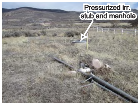
Photo 5. East view of pressurized irrigation stub and manhole observed in the northeast corner of the Project Area. No wetlands or streams observed. Buried pressurized irrigation pipes replaced Wasatch Canal flood irrigation lateral ditch system.
