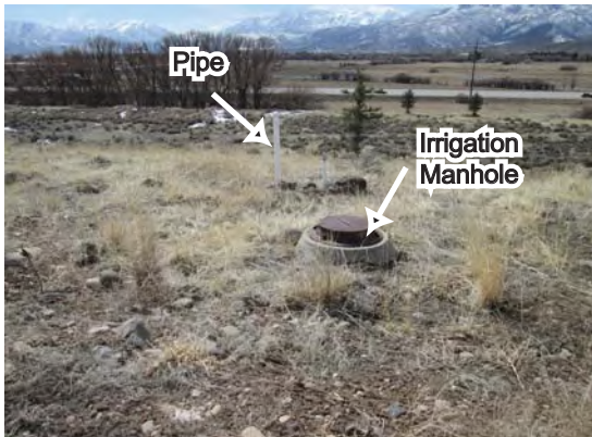
Photo 10. South view of irrigation manhole and stand up pipe stub observed in the northeastern portion of Project Area. No wetlands or streams observed. Pressurized irrigation replaced the Wasatch Canal flood irrigation system.
