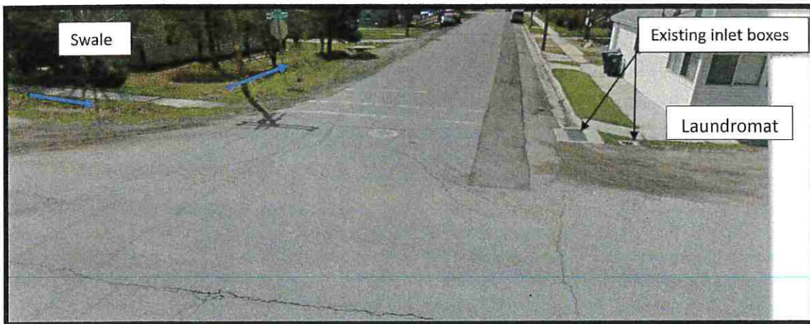
Photo 4 The swale at the intersection of Main Street and 150 South
