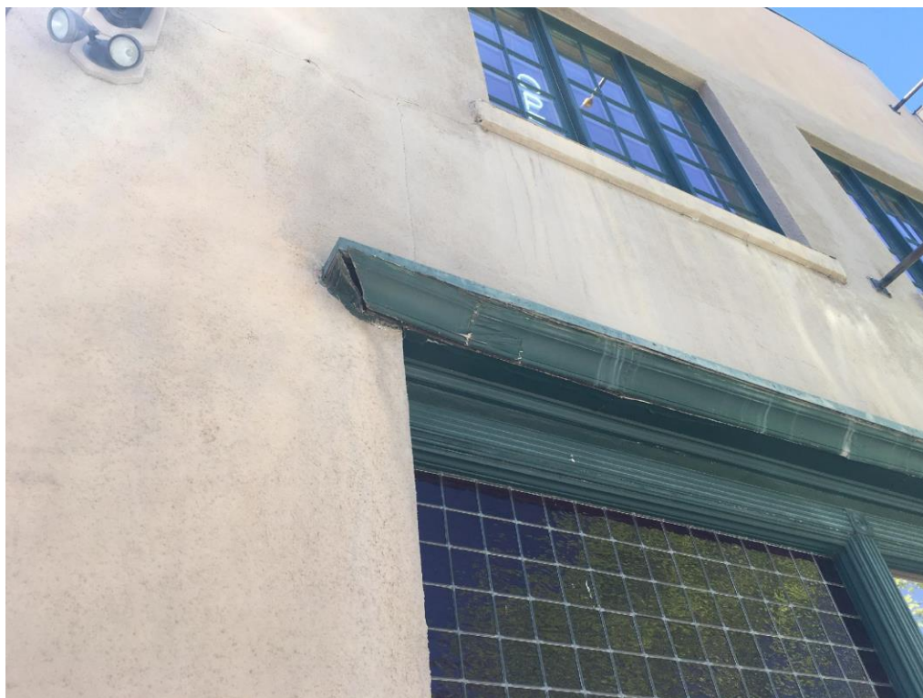
Image 1f (Wooden trim and window pane)
