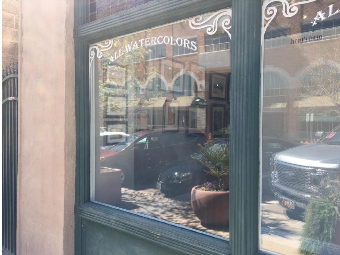
Image 1b (Window pane and current conditions)
