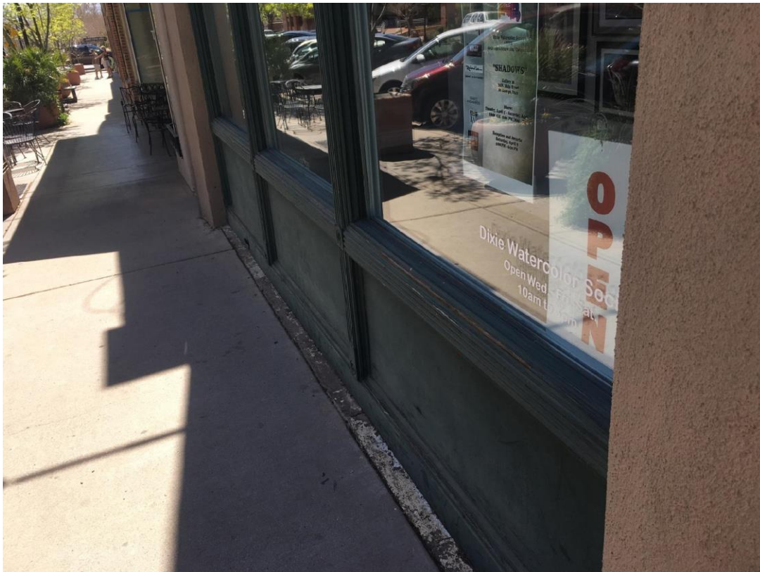
Image 1d (Wooden trim and window pane)
