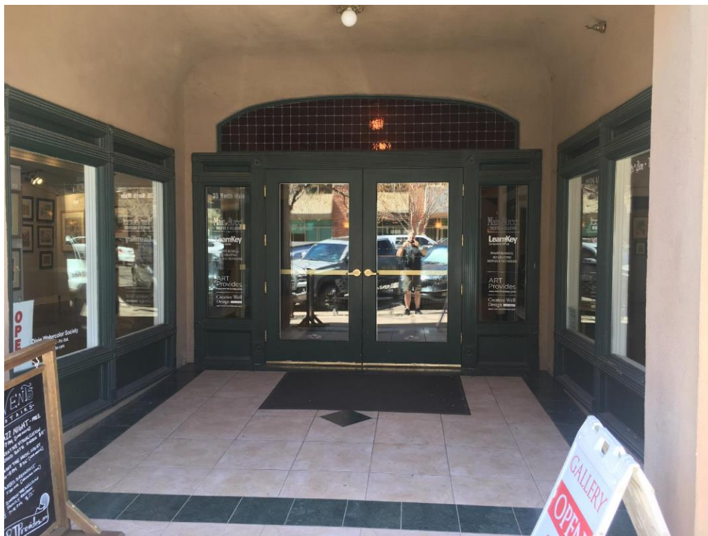
Image 1e (Wooden trim and current conditions)
