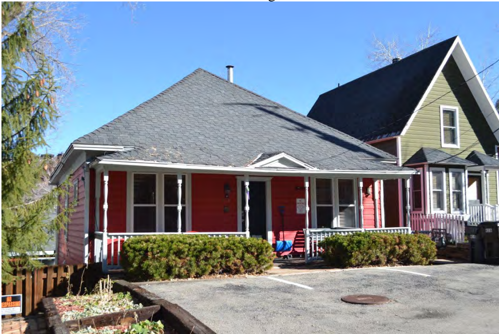
3 of 25. West and north elevations. Camera Facing southeast.
