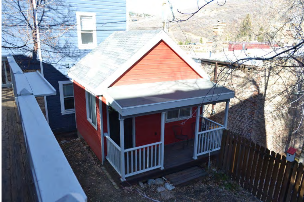
24 of 25. Outbuilding south and west elevations. Camera facing north.
