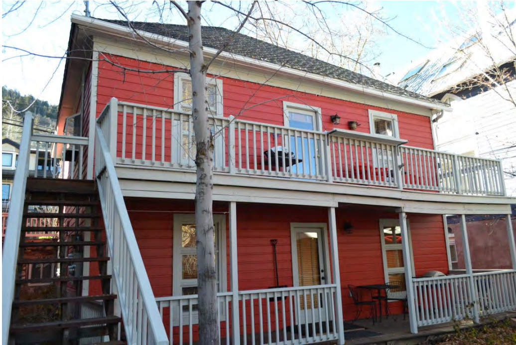
6 of 25. East and south elevations. Camera Facing west.
