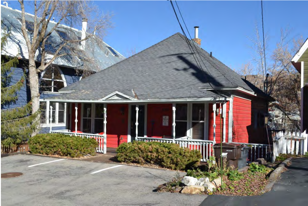
2 of 25. West and south elevations. Camera Facing northeast.
