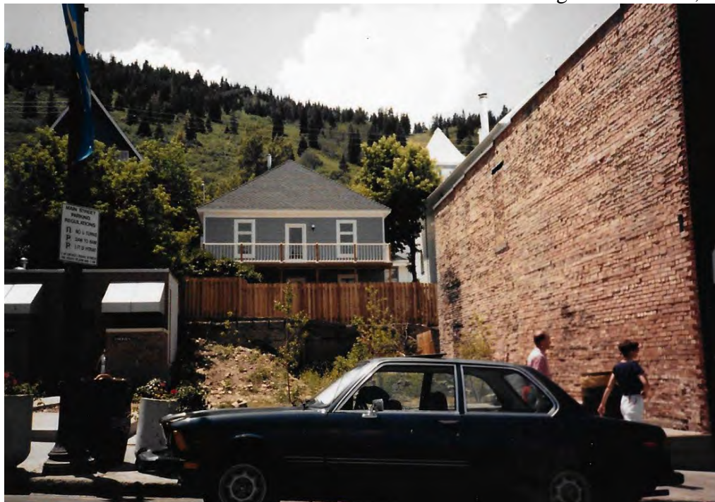
Figure 5. 416 Park Avenue east elevation from Main Street following rehabilitation, 1988.
