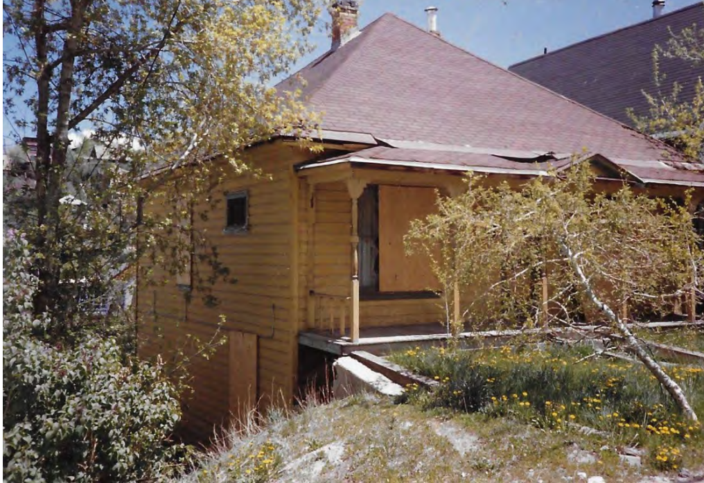
Figure 3. 416 Park Avenue north and west elevations prior to rehabilitation, 1988.
