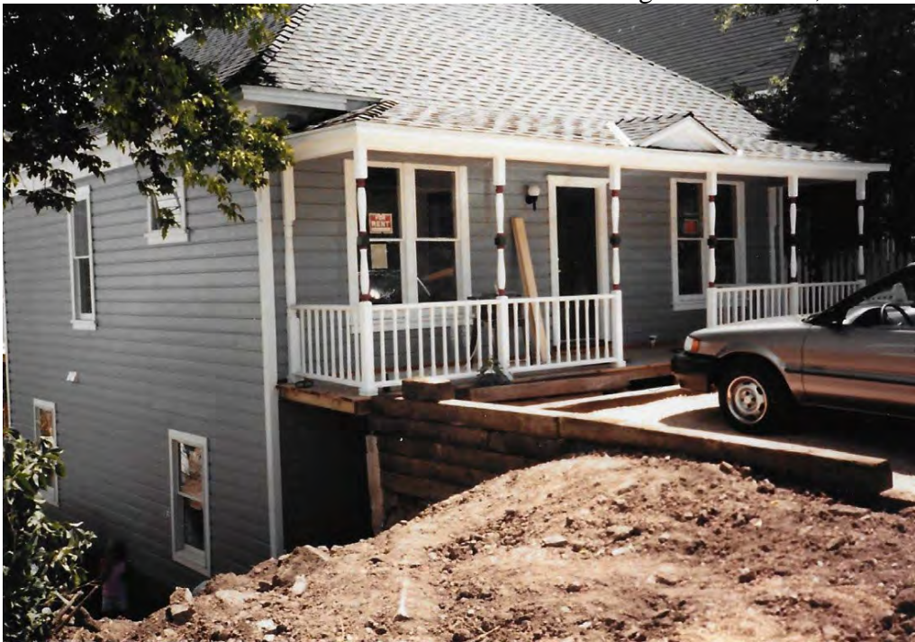
Figure 4. 416 Park Avenue north and west elevations following rehabilitation, 1988.
