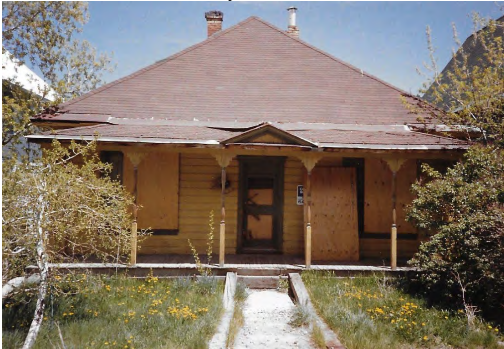
Figure 2. 416 Park Avenue west elevation prior to rehabilitation, 1988.
