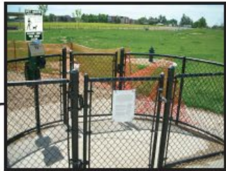
Double gate entry systems (4 Entries)
