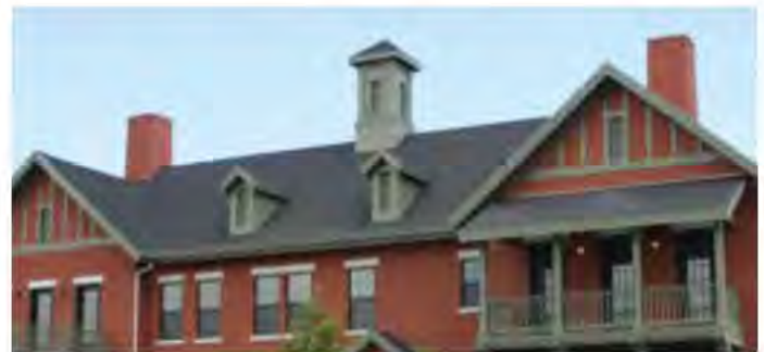
Roof Materials: Asphalt Composite Shingles
