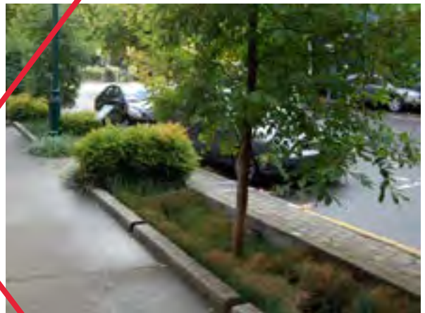
Figure 2.3 (4). Curb Cut and Landscape Storm Drainage Methods
