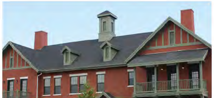
Roof Materials: Asphalt Composite Shingles
