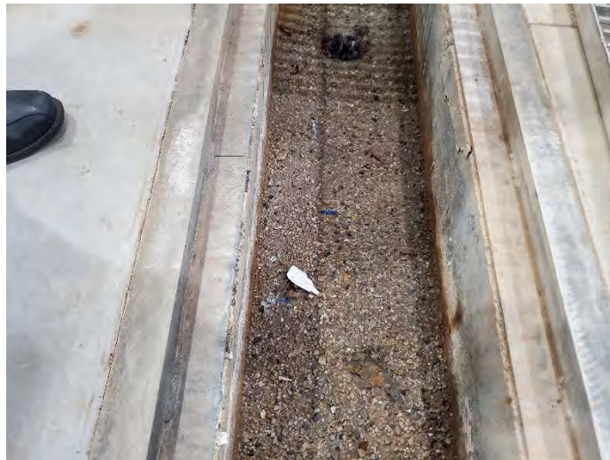
Figure 3 - Drainage Trough, Concrete Damage
