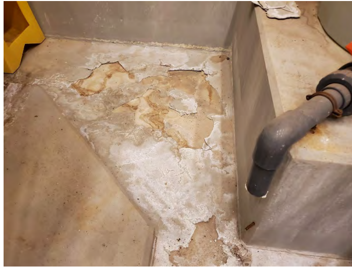
Figure 2 - Concrete Coating Failure
