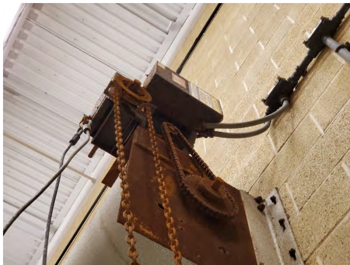
Figure 5 - Exposed Steel on the Overhead Door System
