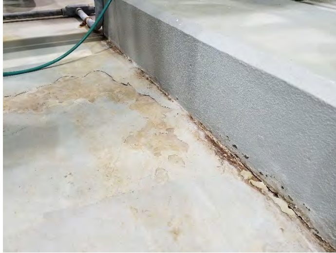
Figure 4 - Coating Failure from Improper Surface Preparation
