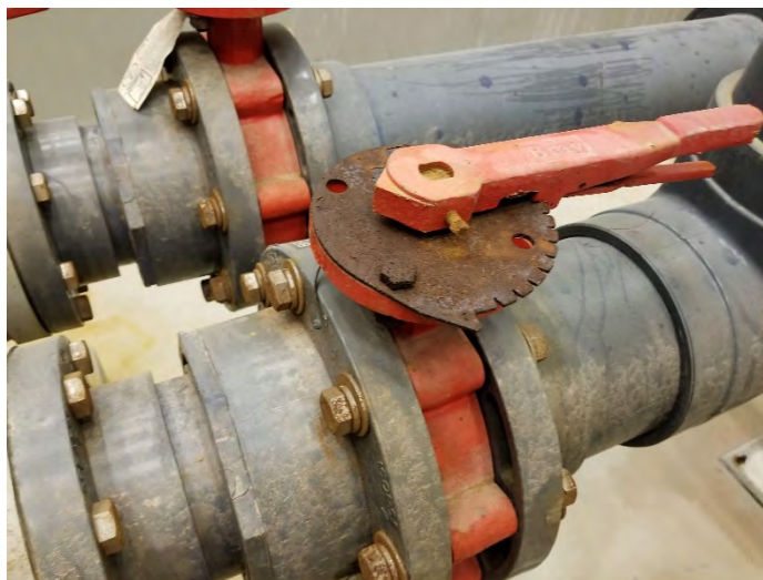
Figure 8 - Stainless Steel Bolts on a Flanged Connection
