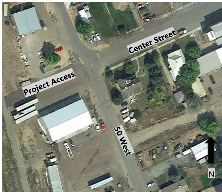
Figure 1: Project Site Area (images courtesy of Google Earth)
