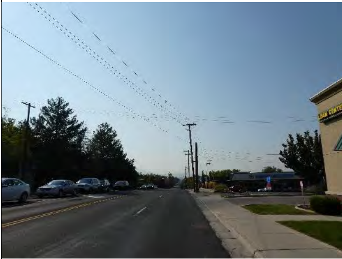
Street View: 1300 East Looking Southerly (Site is at Right)
