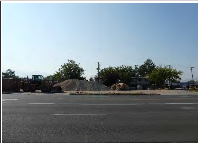
Looking Southerly Across Site
