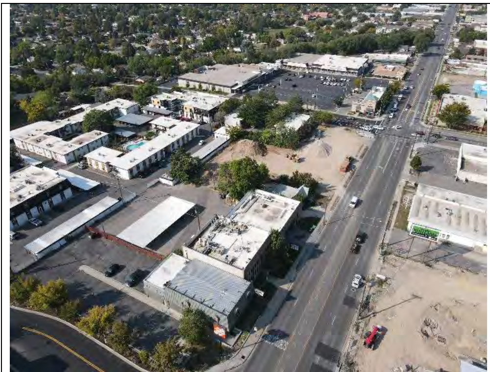
Looking Southwesterly at the Site
