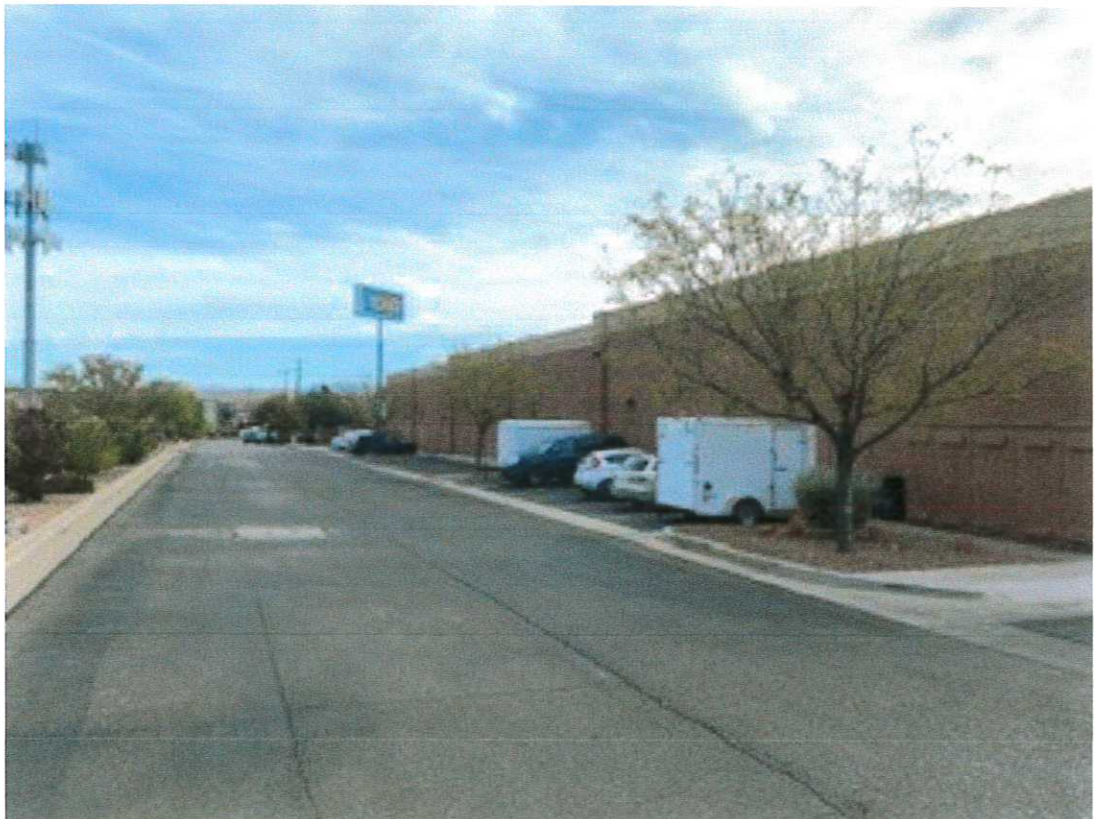
BACK OF Building
