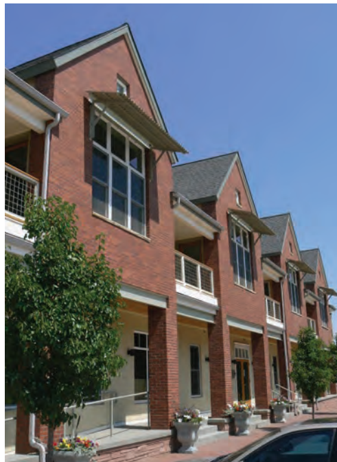
Forward facing gables, awnings, covered balconies create an appealing composition together with the ground floor colonnade.
