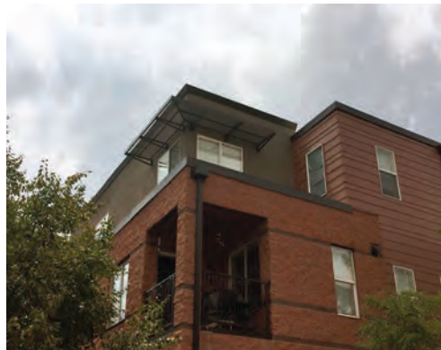
Uppermost story setbacks such as the one shown here create appealing horizon lines on the corners.
