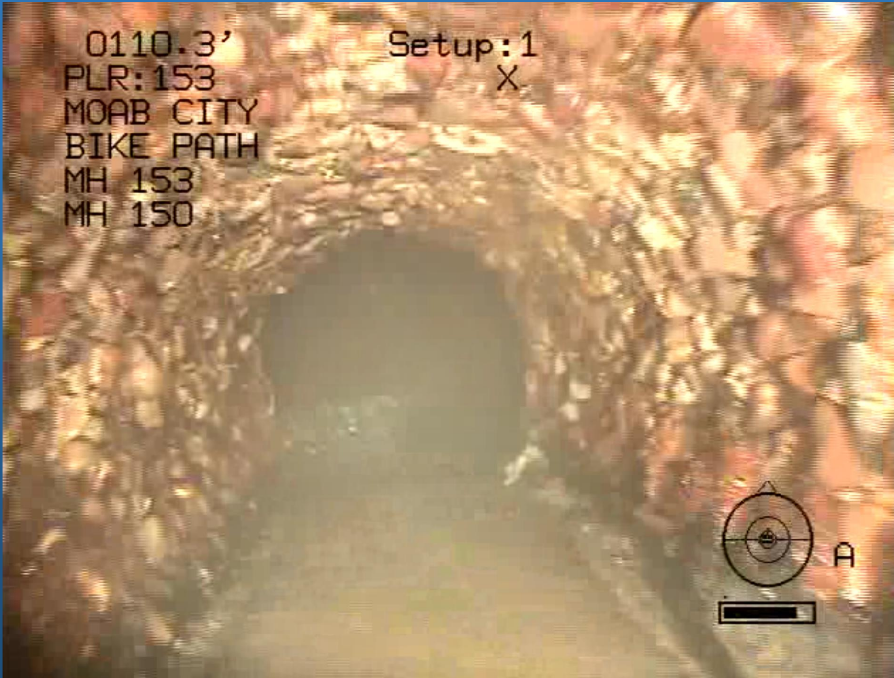
100 West pipe under Mill Creek
