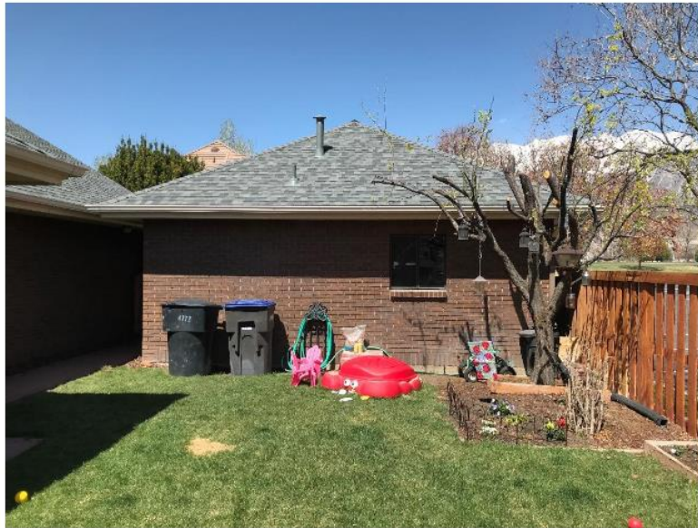
Photo #1: Looking northward at the south end of the existing garage showing the 18" setback from the fence and property line on the east side of our property.
