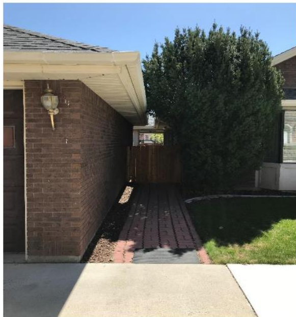
Photo #8: Southward view from site of proposed new garage showing existing house on the right and the walkway separating house from unattached existing garage which we hope to repurpose.
