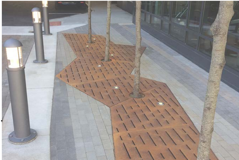
DECORATIVE TRENCH GRATE
