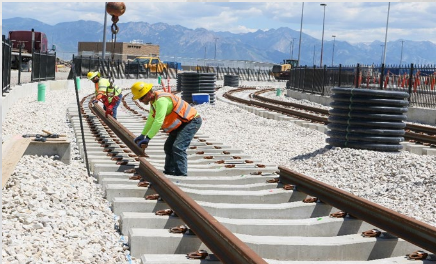
TRAX Line Installation
