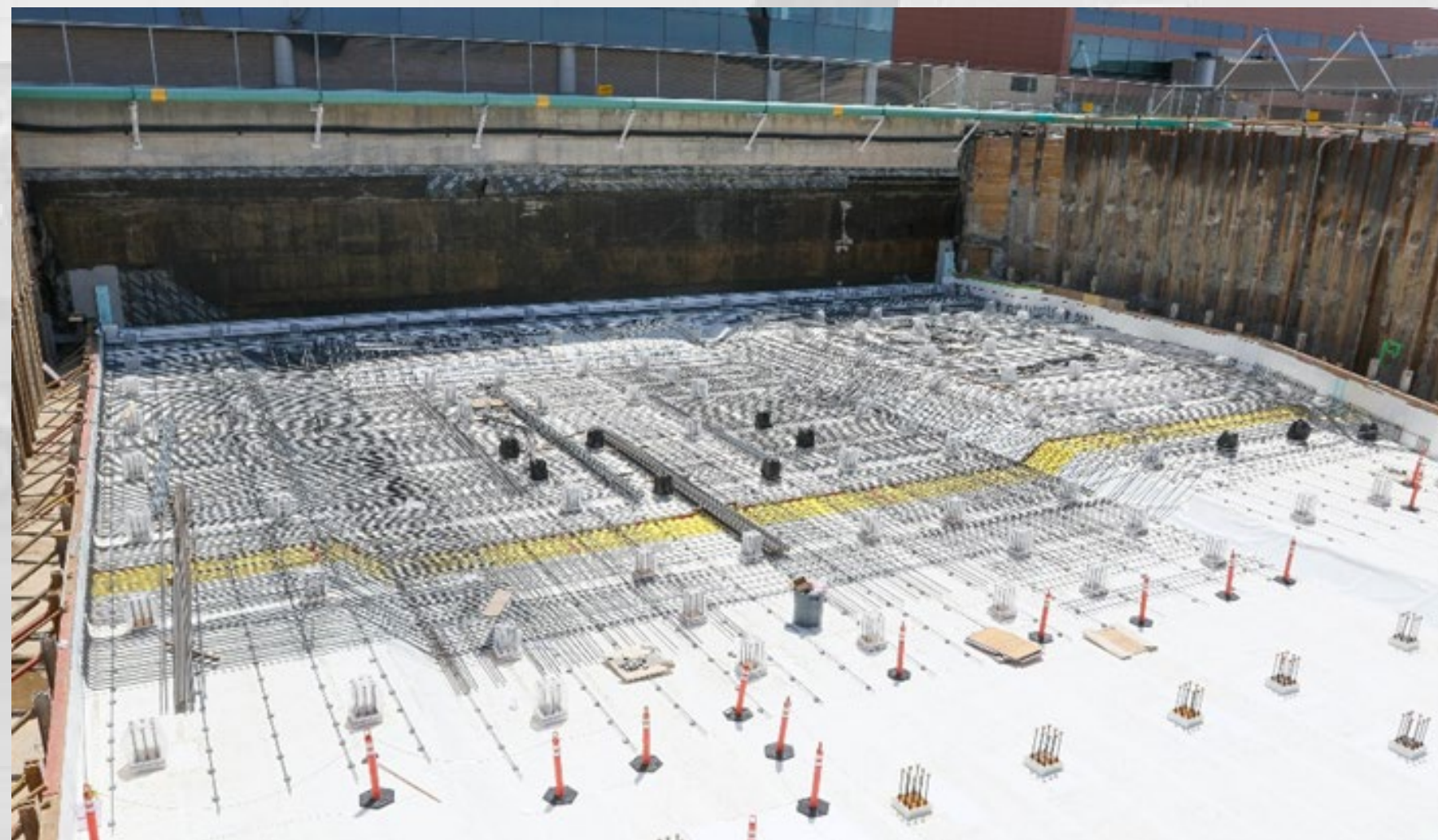
Bottom Slab Reinforcing Steel
