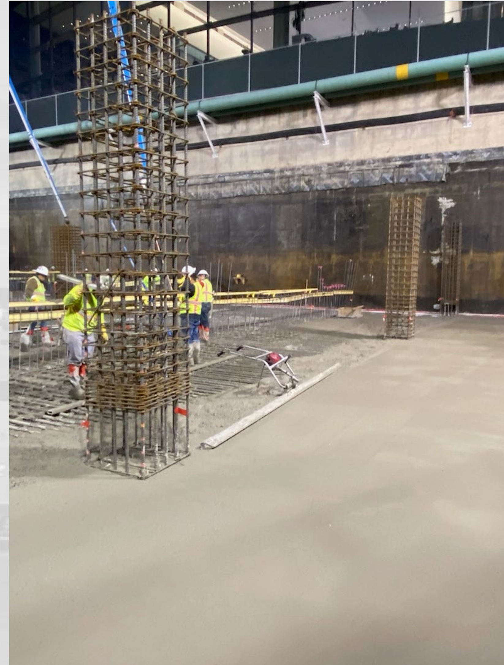
First Bottom Slab Concrete Placement 1,455 cy
