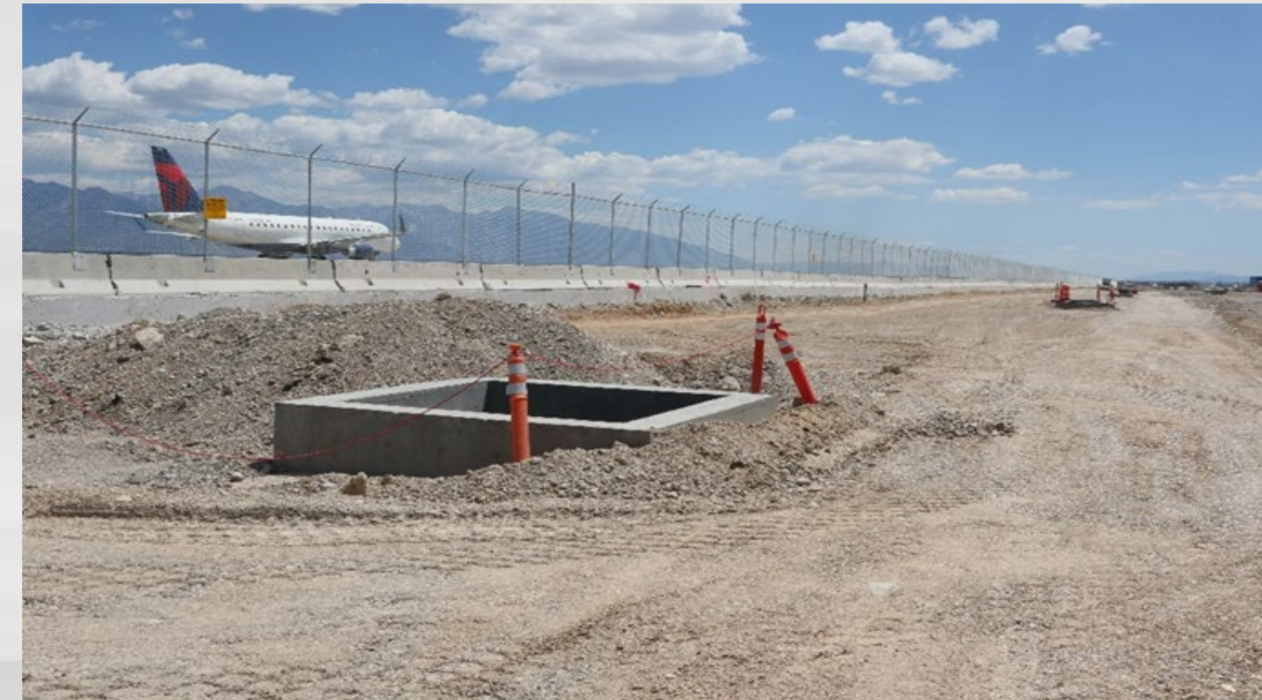
60" Storm Line Backfill & Grading
