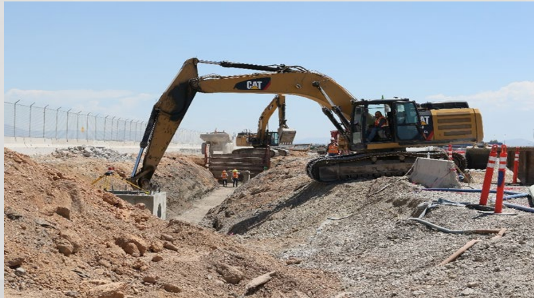
60" Storm Line Installation
