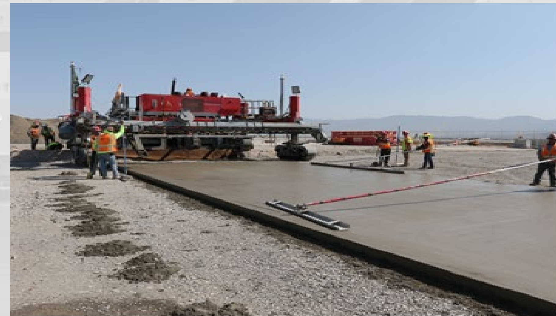
Lean Concrete Placement
