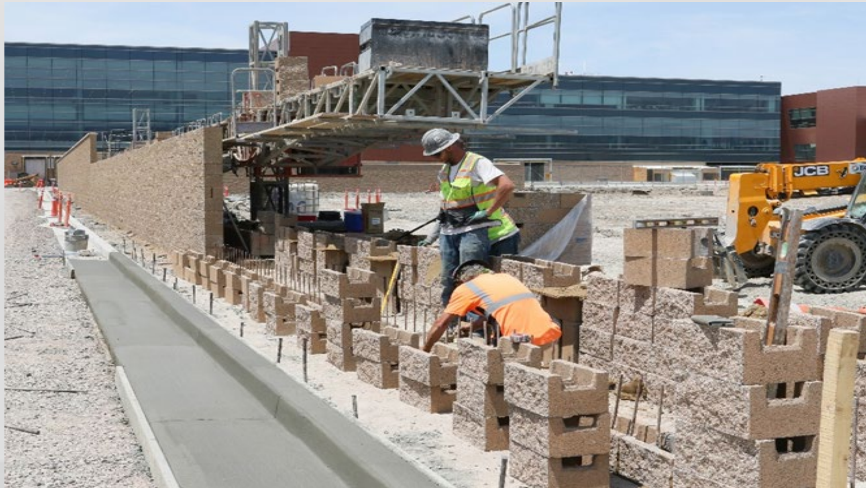
AOA Wall Near TRAX Line
