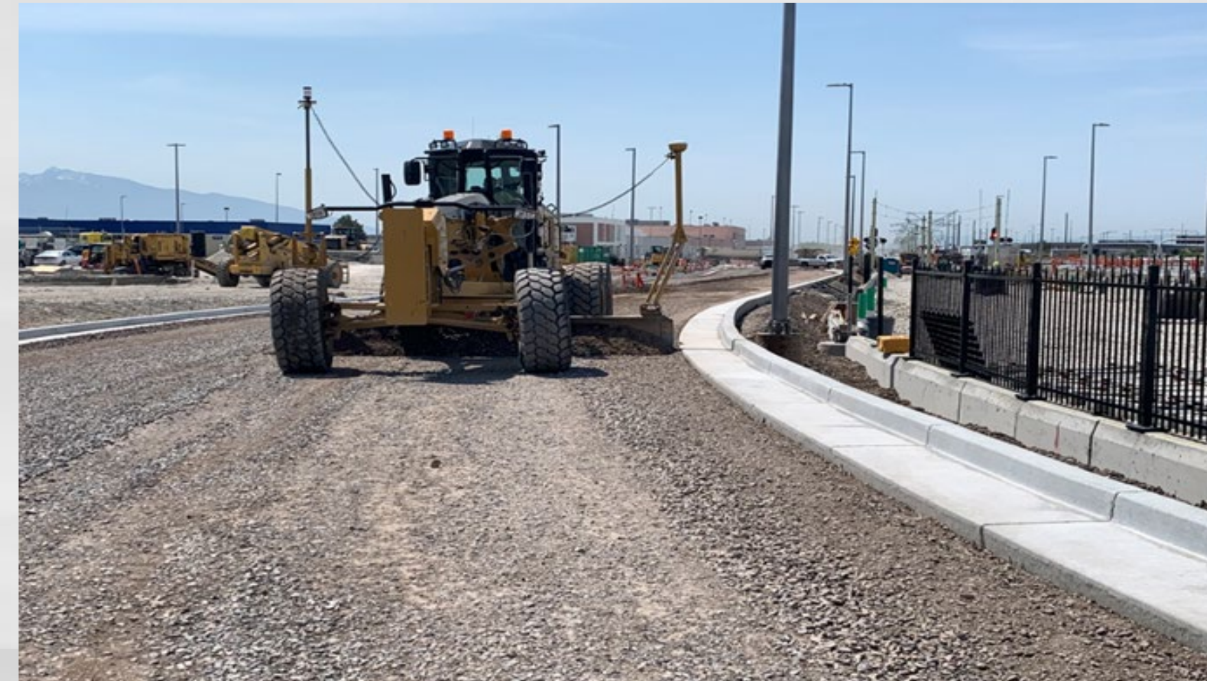
3700 W / Cargo Road Grading
