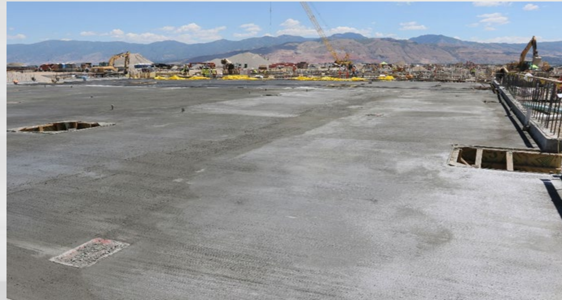
Slab on Grade Placement
