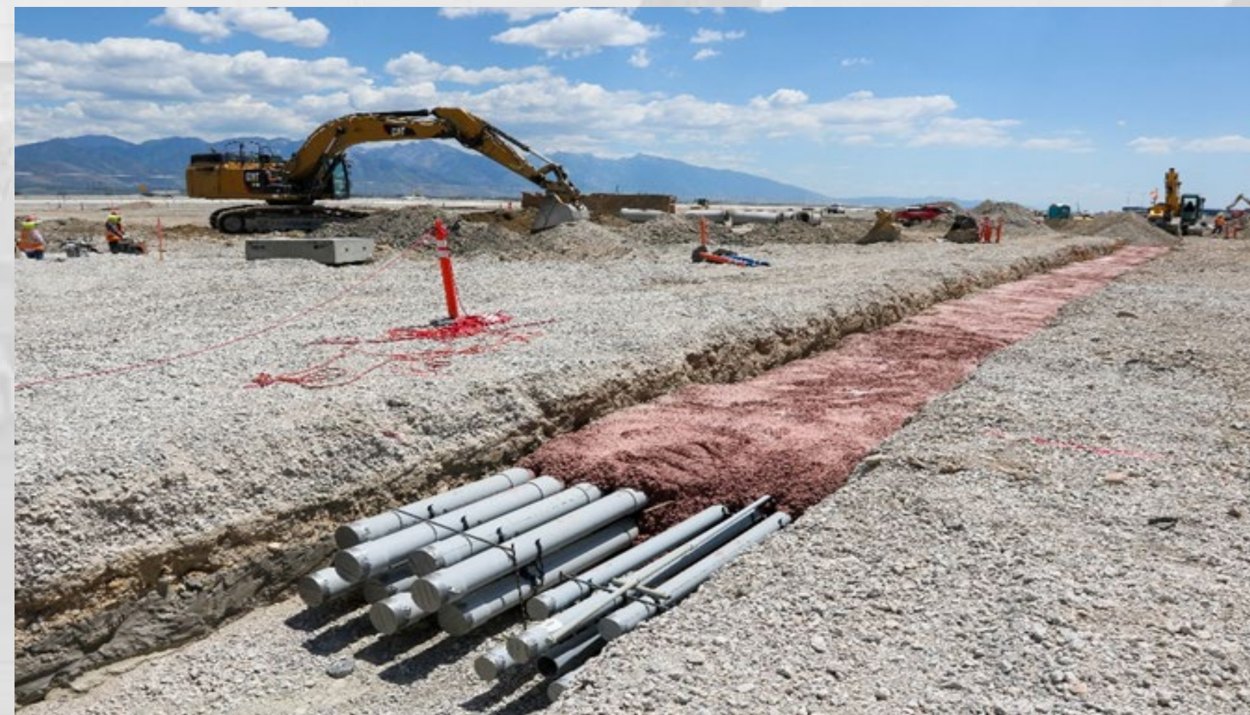
Electrical Ductbank Installation
