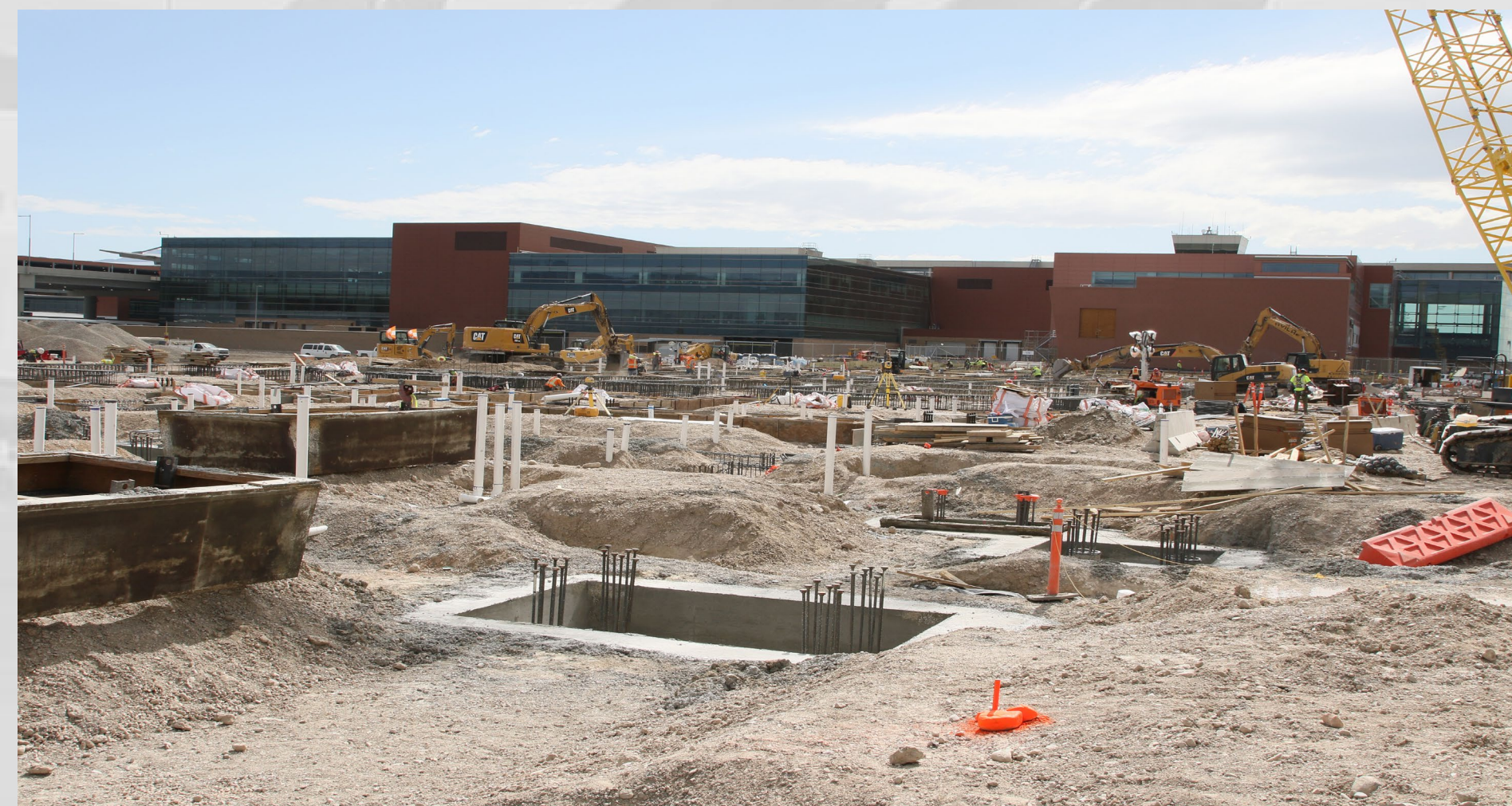
Pile Caps and Shallow MEP
